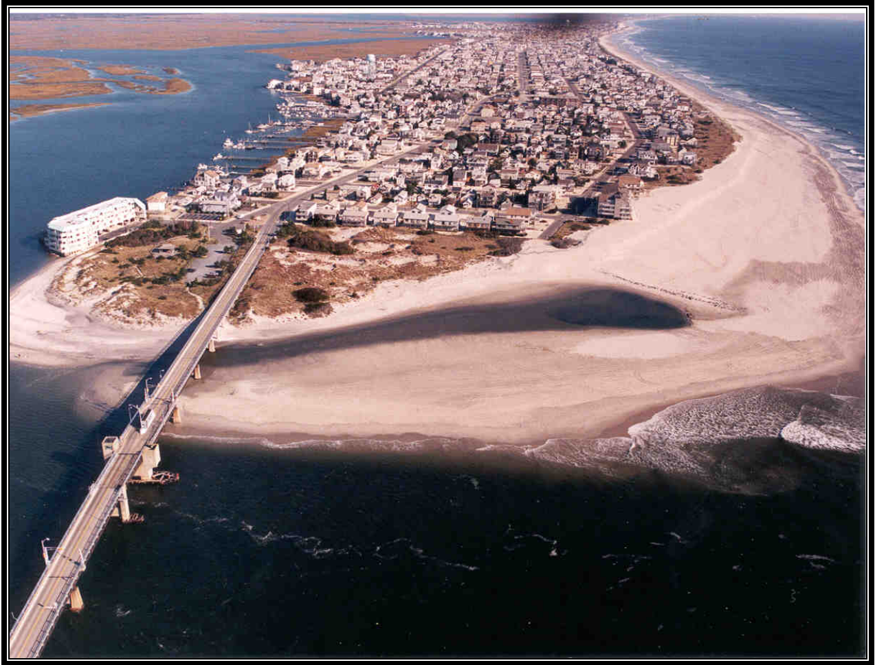
Photo 1-11 Townsends Inlet area of Sea Isle City, NJ, 10/25/99. Following construction of terminal groin and beachfill placement by locals.
