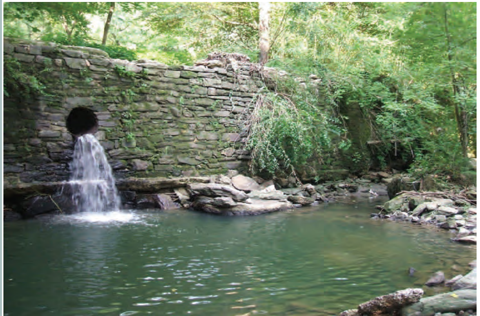
Upstream view of Cresheim Dam
