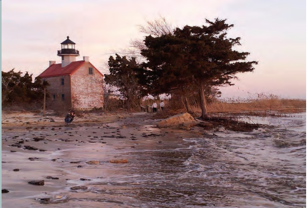
East point Lighthouse in the background with rapidly Eroding marsh in the foreground.
