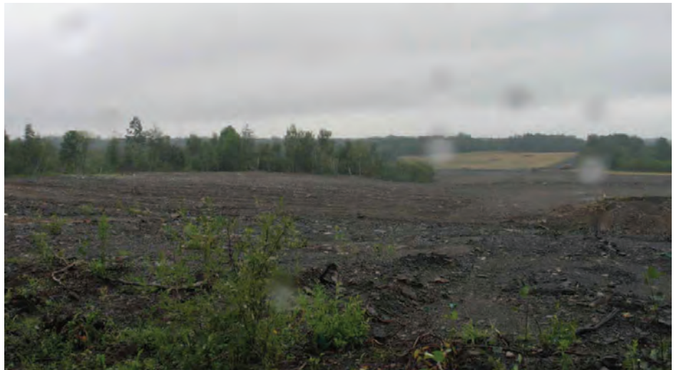
Hazelton Area Mine Reclamation Site
