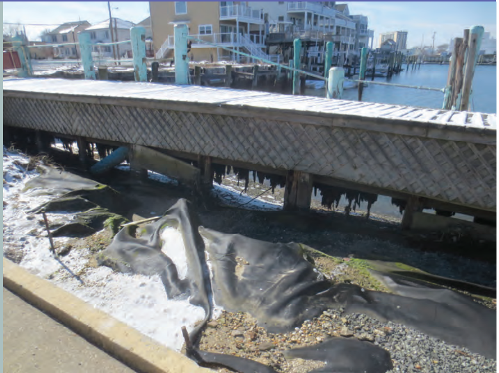
The photo above shows the deteriorated condition of the Bulkhead at Massachusetts Avenue in Atlantic City.
