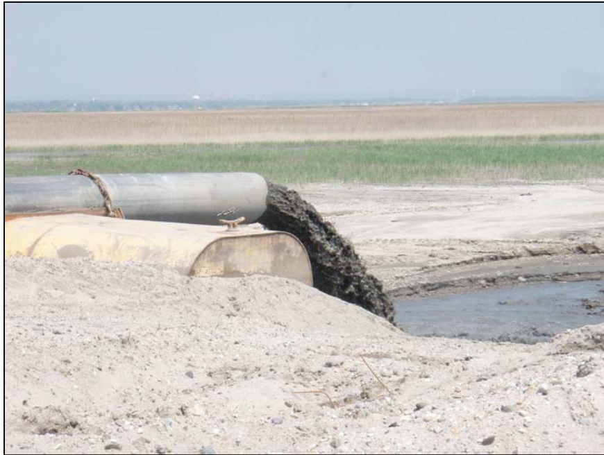
Figure 6-3. Dredged slurry being pumped into a typical CDF along the banks of the Delaware River
