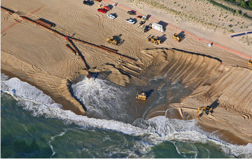
Figure 10. A Typical Beachfill Operation along the Delaware Atlantic Coast. (Source: Great Lakes Dredge and Dock Company website accessed at: http://www.gldd.com/company/projects/coastal-protection/ on 5/7/2015)
