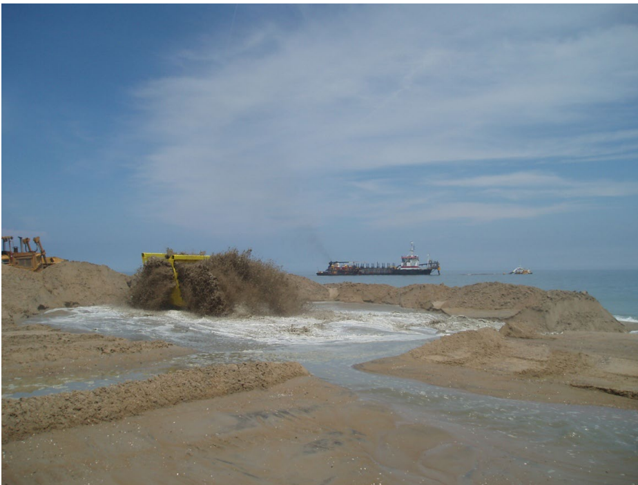
Figure 11. Sand Being Pumped Through a 3/4-inch MEC Screen Basket from a Hopper Dredge. Training berms surround pump-out area to allow for sand retention.
