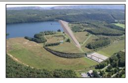
feet wide with a crest elevation of 651 feet NAVD 29. The spillway can release up to 368,016 gallons per second or approximately one-half the volume of an Olympic-sized swimming pool each second. The earthen dam is 4,560 feet long and 170 feet high, and the top of the dam is 30 feet wide. The elevation of the top of the earthen embankment is 672 feet NAVD 29. The foundation consists of shale and sandstone bedrock.
