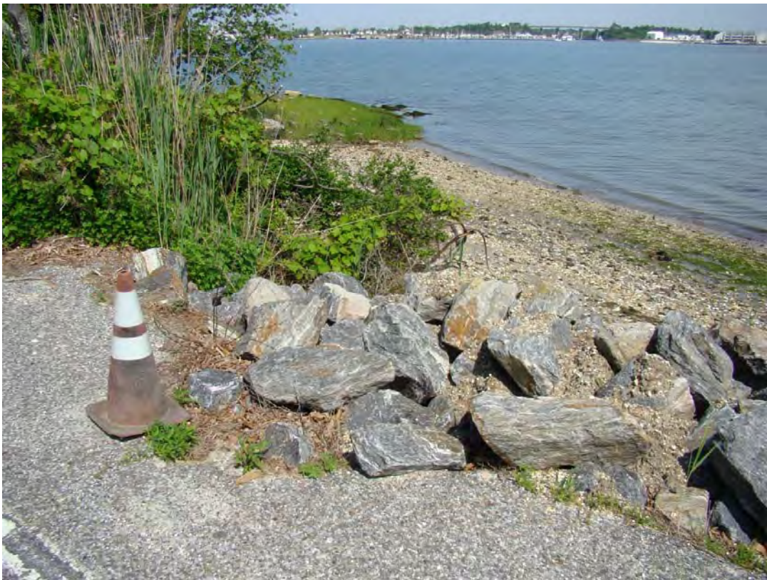
Photograph 4: Looking west at emergency rip-rap placed following Hurricane Sandy at Wilmington Avenue.
