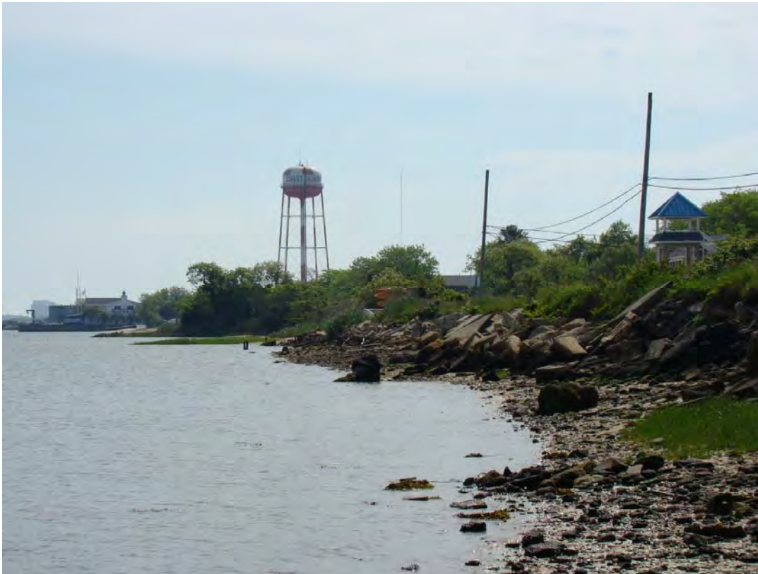
Photograph 2: Looking east along the shoreline from Brooklyn Avenue.
