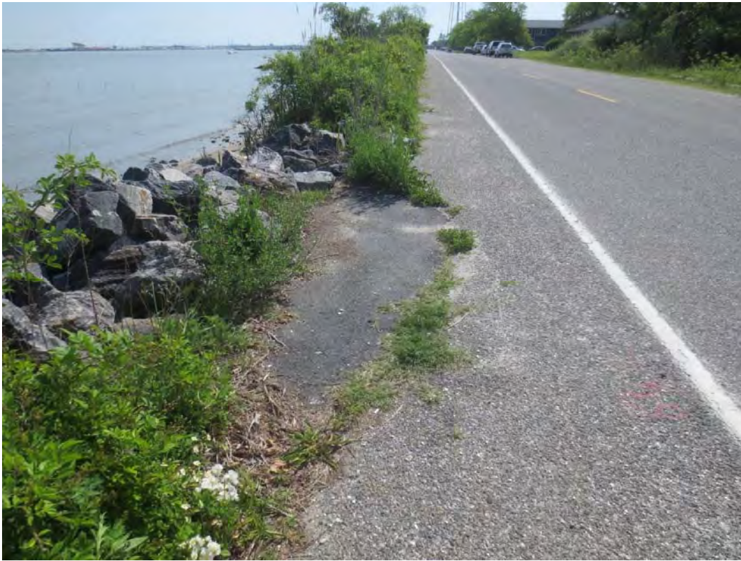
Photograph 3: Looking northeast at an asphalt patch and emergency rip-rap that was placed following Hurricane Sandy between Brooklyn and Wilmington Avenues.
