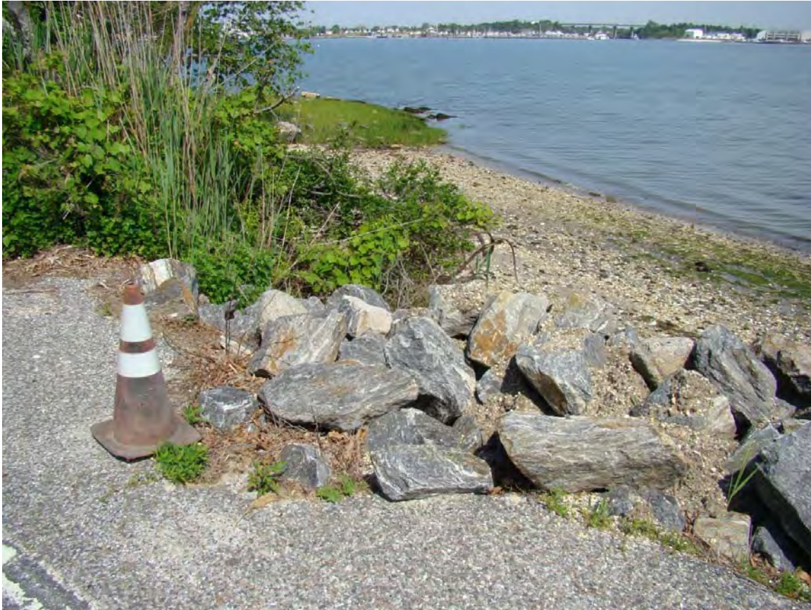
Figure 5: Emergency rip-rap placement area following Hurricane Sandy.
