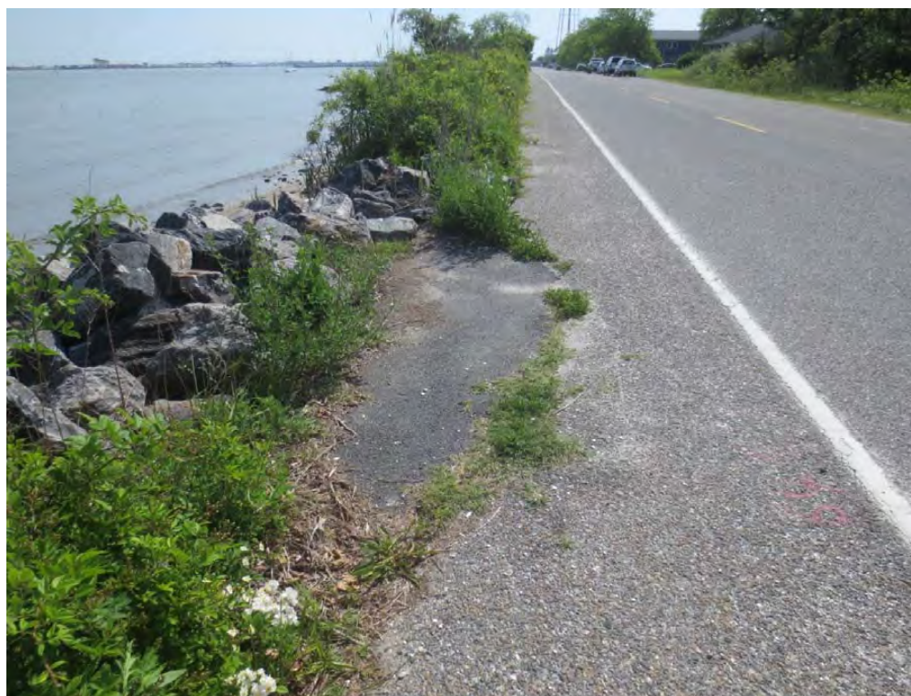
Figure 4: Asphalt patch and emergency rip-rap placement area following Hurricane Sandy.
