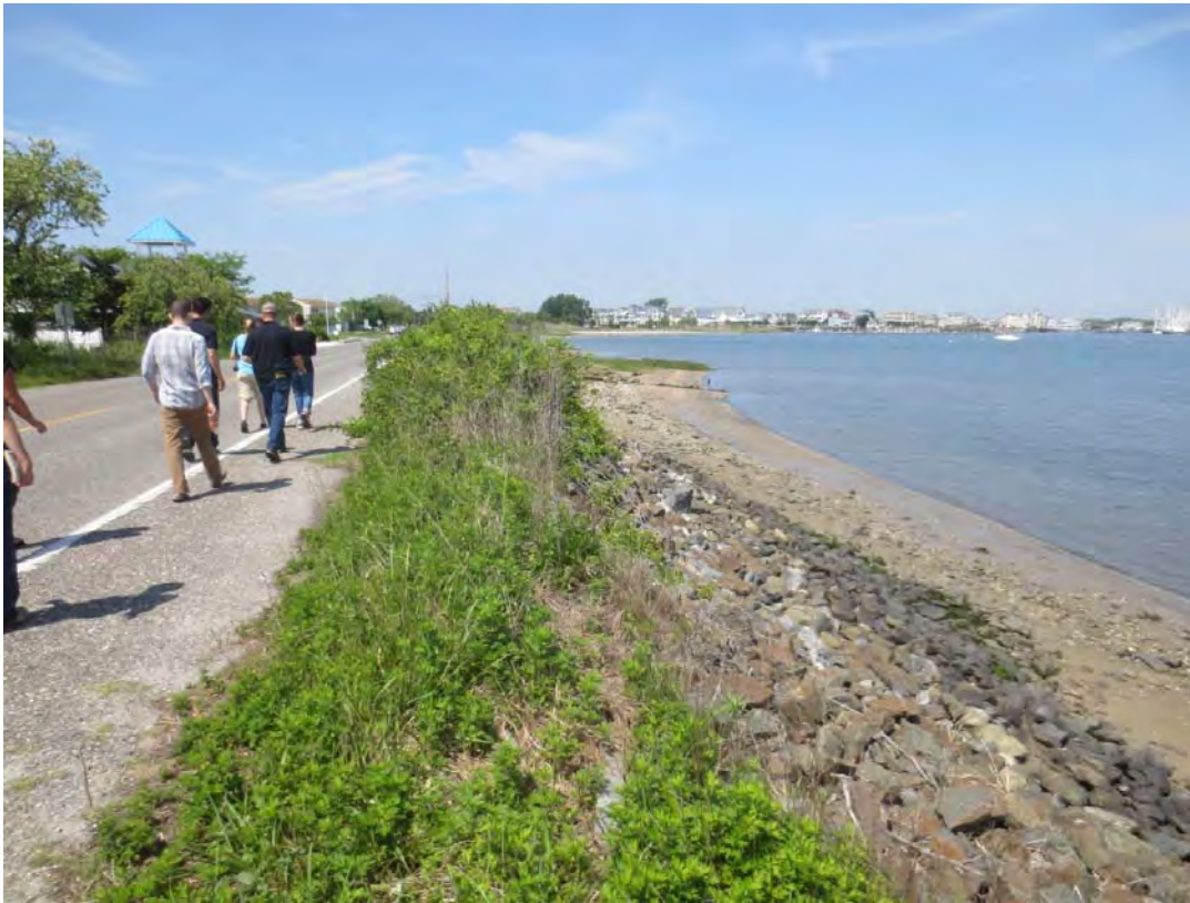
Photograph 1: Looking southwest along Delaware Avenue between Brooklyn and Wilmington Avenues.
