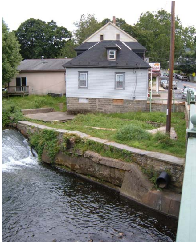
Photograph 4 – Southern embankment of the dam and the adjacent residential property in Borough of Bloomsbury.
