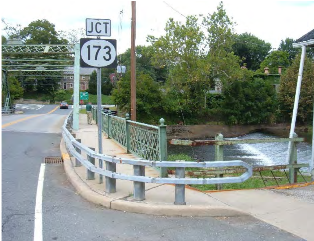
Figure 4. Dam and downstream bridge on Route 579 (Church Street).
