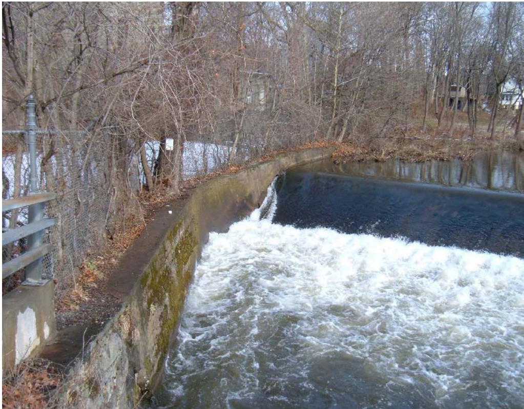
Photograph 5 – Northern embankment of the dam in Greenwich Township.
