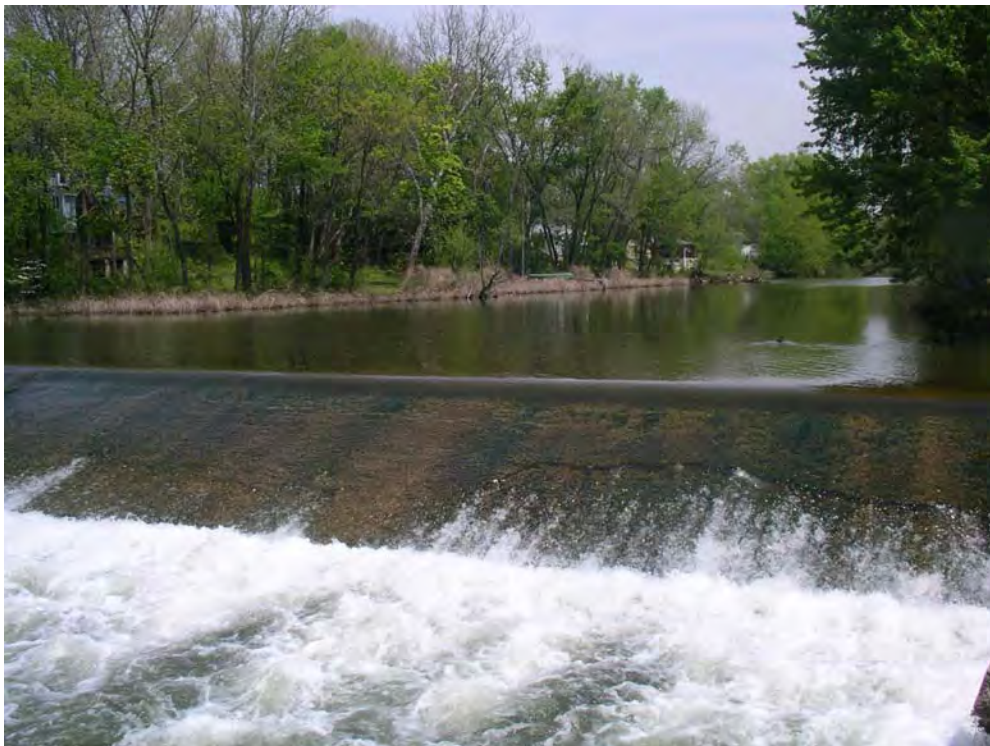
Upstream view of Bloomsbury Dam
