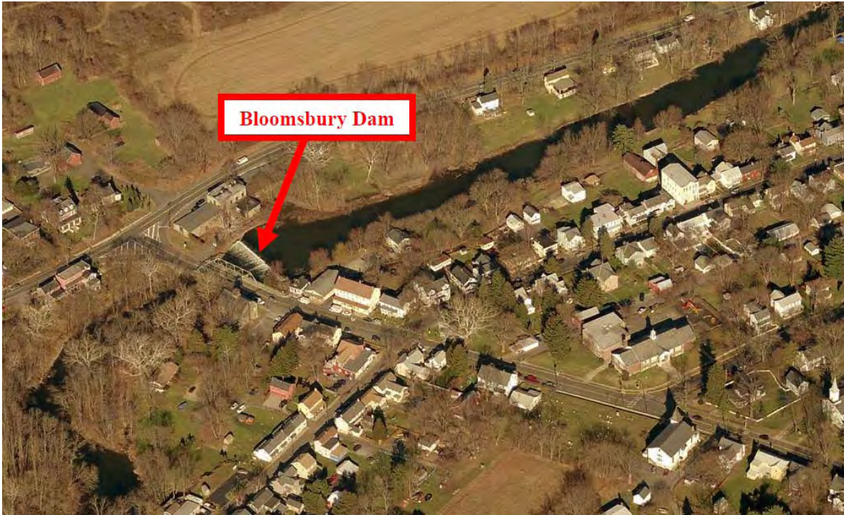
Figure 2. Bloomsbury dam aerial photograph.
