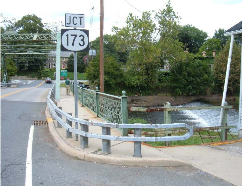
Photograph 2 – Dam and downstream bridge on Route 579 (Church Street).
