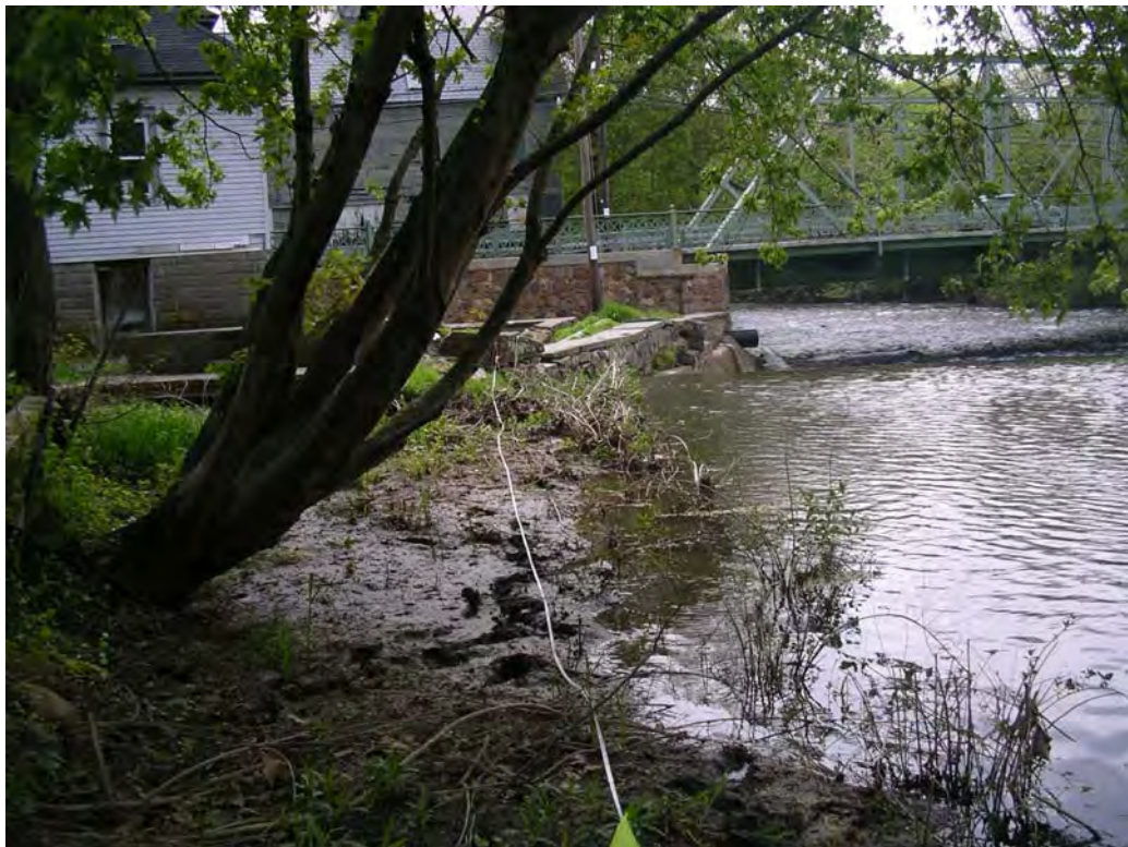
Left bank of Bloomsbury Dam looking downriver from impoundment
