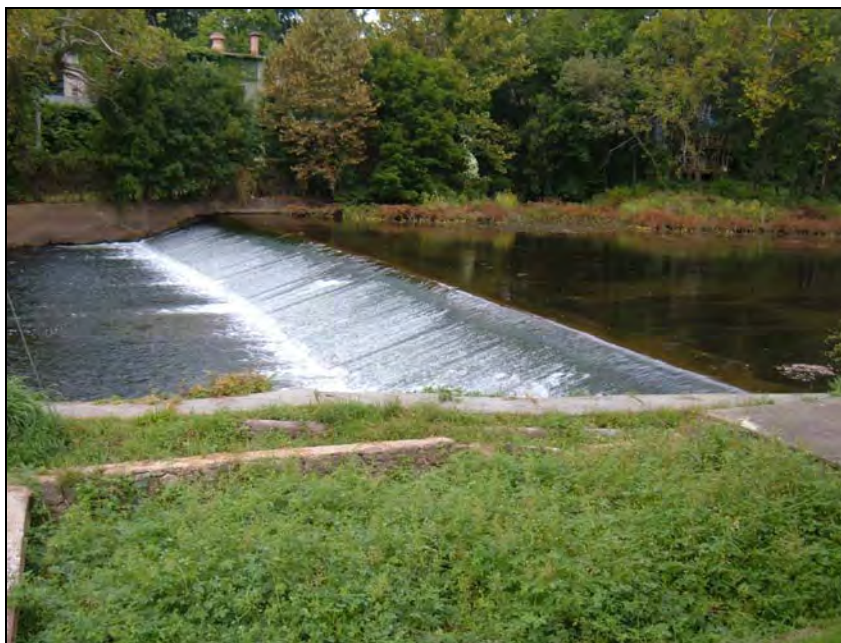
Figure 1-2. Bloomsbury Dam shown from the southern bank in Hunterdon County, NJ (Photo date: September 2009).
