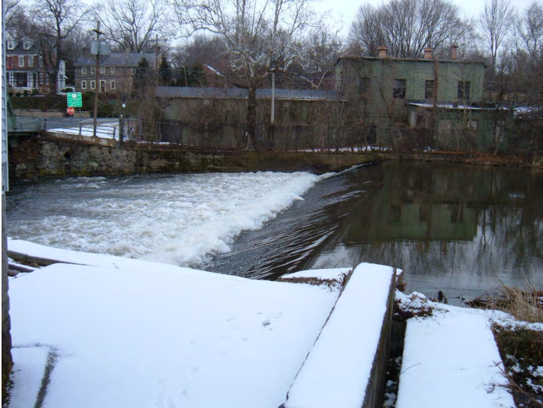
Figure 6. Former industrial facility adjacent to the dam on north riverbank.
