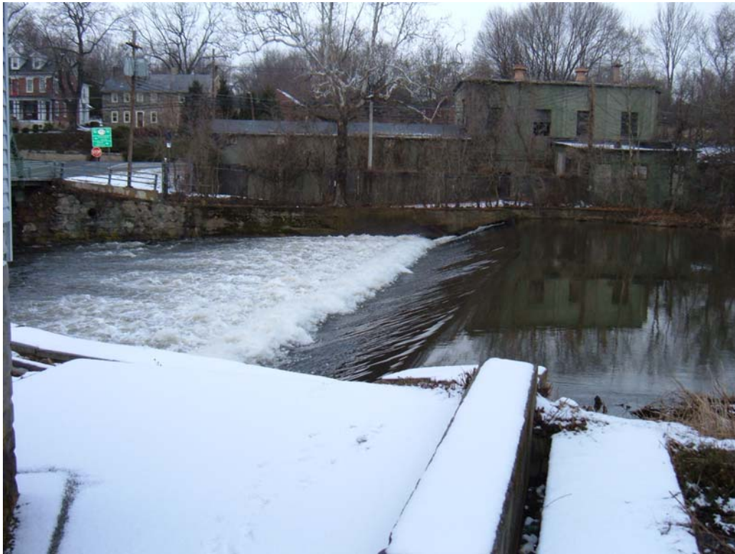
Photograph 6 – Former industrial facility adjacent to the dam in Greenwich Township.
