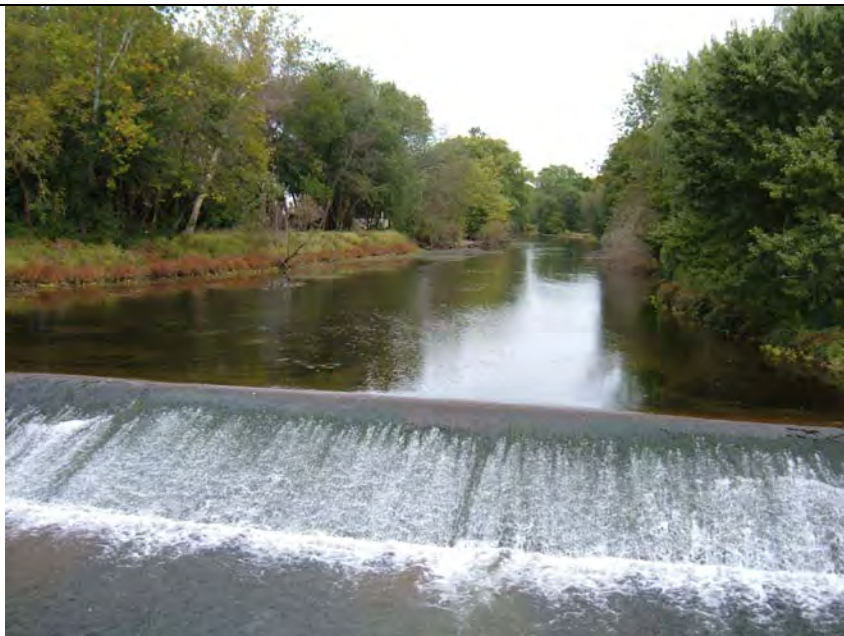
Figure 3: Bloomsbury Dam and the upstream impoundment shown from the Church Street bridge (County Road 579) approximately 90 feet downstream of the dam. Photo taken September 10, 2009.
