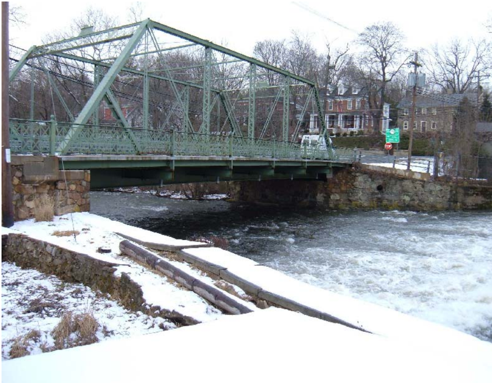
Photograph 3 – Downstream bridge on Route 579 (Church Street).
