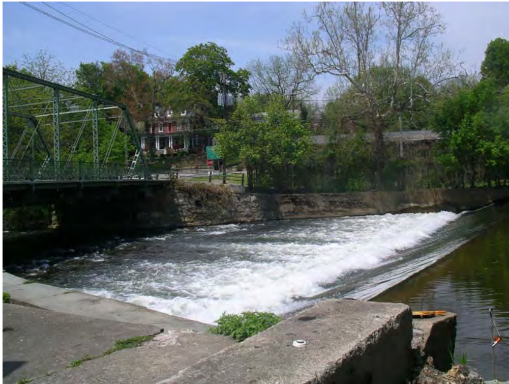
Left bank of Bloomsbury dam looking downriver at dam crest
