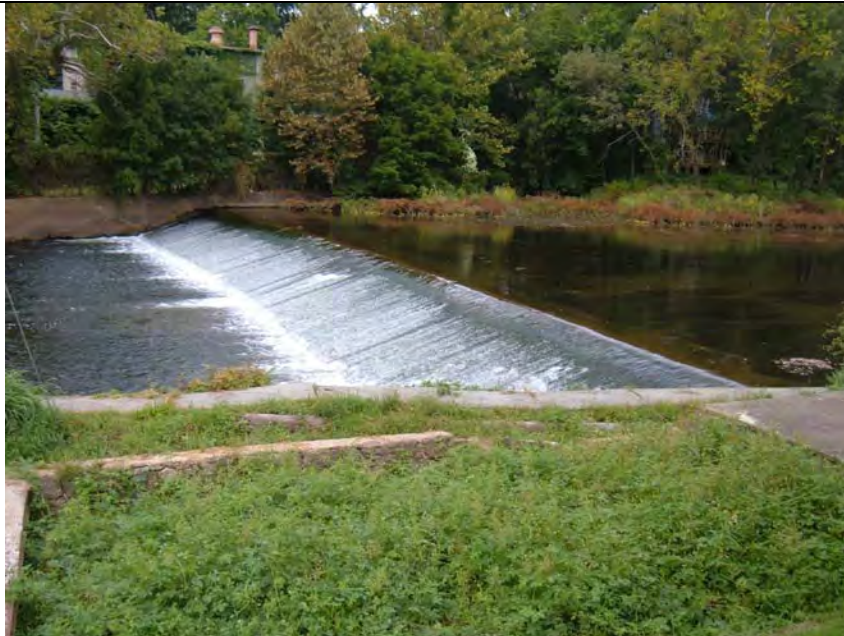
Figure 2: Bloomsbury Dam shown from the southern bank in Hunterdon County. Photo taken September 10, 2009.
