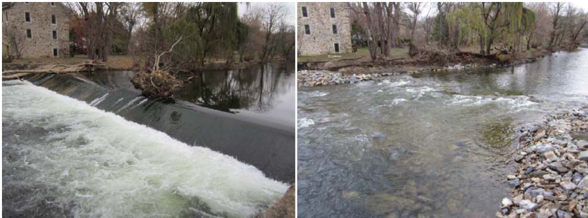
Figure 6 – Finesville Dam Before and After Removal
