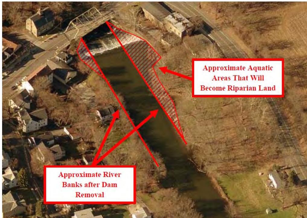
Figure 7. Estimated change in river width in Bloomsbury, as a result of dam removal.
