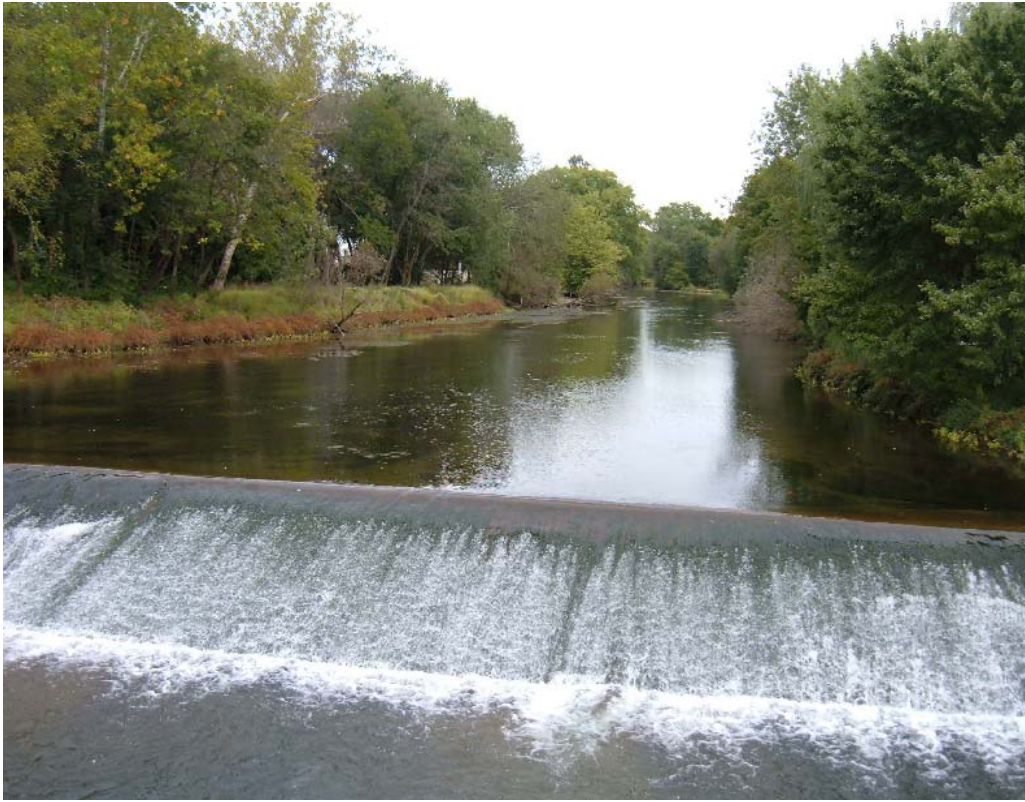
Photograph 8 – Impoundment upstream of the Bloomsbury Dam.
