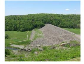
dam that maintains no pool during normal operation. The dam can provide 24,500 acre-feet of storage up to the spillway crest and a total of 47,300 acre-feet of storage at maximum pool.
