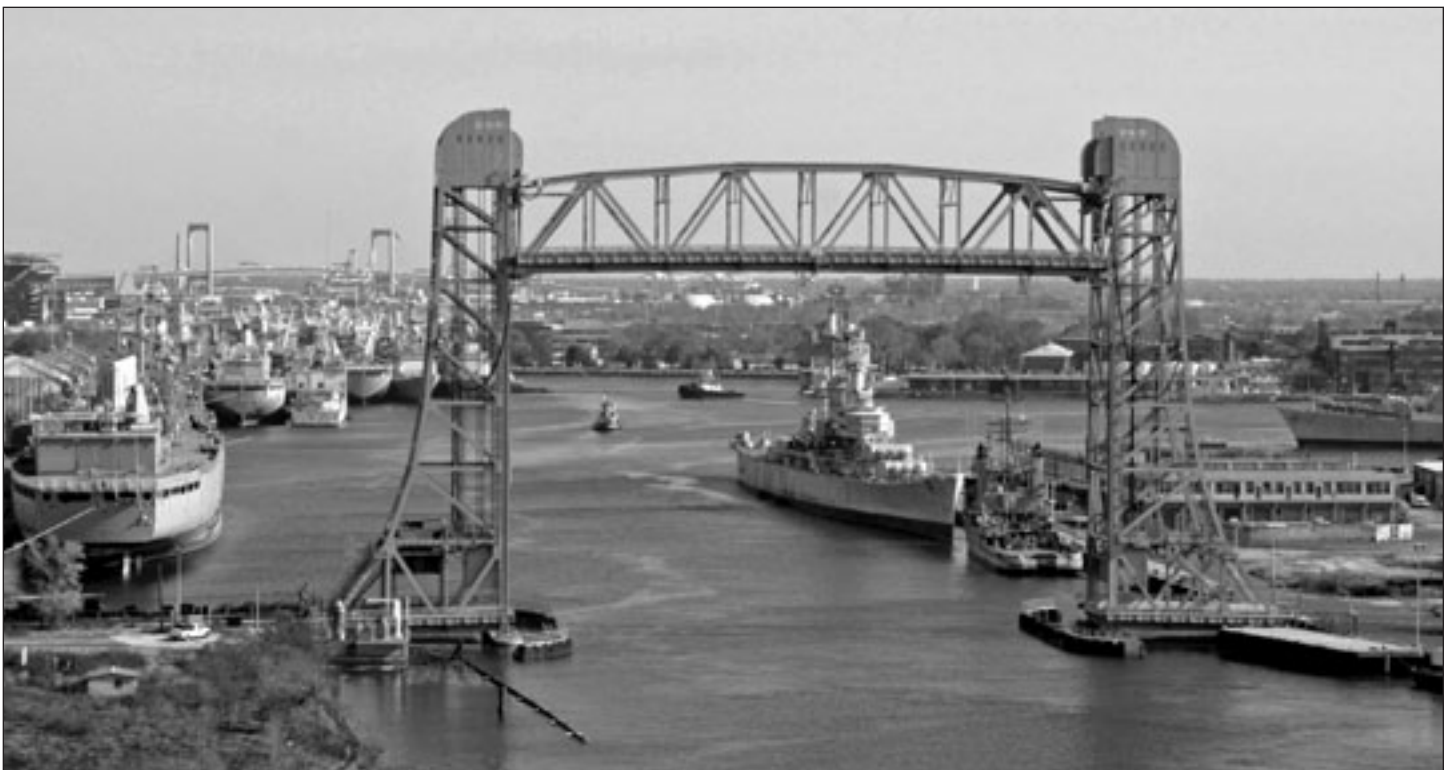
The vertical lift bridge at the former Philadelphia Naval Shipyard, after complete renovation by the District for the United States Coast Guard
