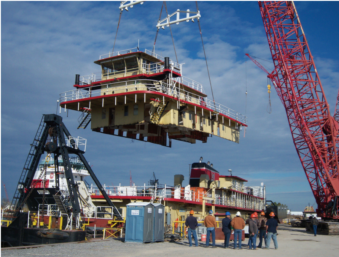
Original deckhouse being lifted off Dredge Potter
