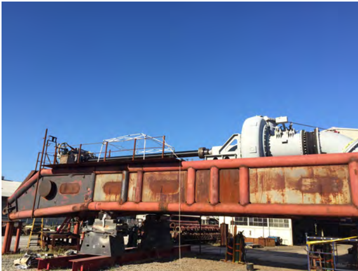
Dredge HURLEY Ladder Extension under construction
