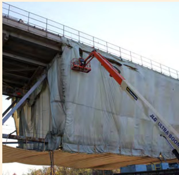
Workers for contractor Marinis Brothers, Inc. perform below-deck repairs.
