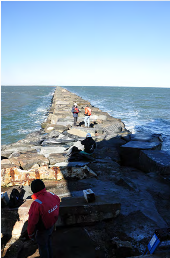
Above: The Corps completed repairs to the Harbor of Refuge breakwater in December. The project involved placing 91 capstones. Top right: The historic lighthouse sits atop the breakwater.
