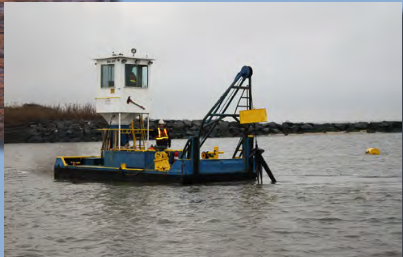
Above: Southwind Dredging Company employees adjust subline as part of a dredging project in the New Jersey Intracoastal Waterway.
