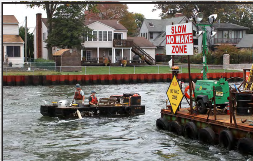
The U.S. Army Corps of Engineers Philadelphia District and its contractor Abhe & Svoboda Inc. use a barge as a staging area during repair work of the Point Pleasant Canal bulkhead.
