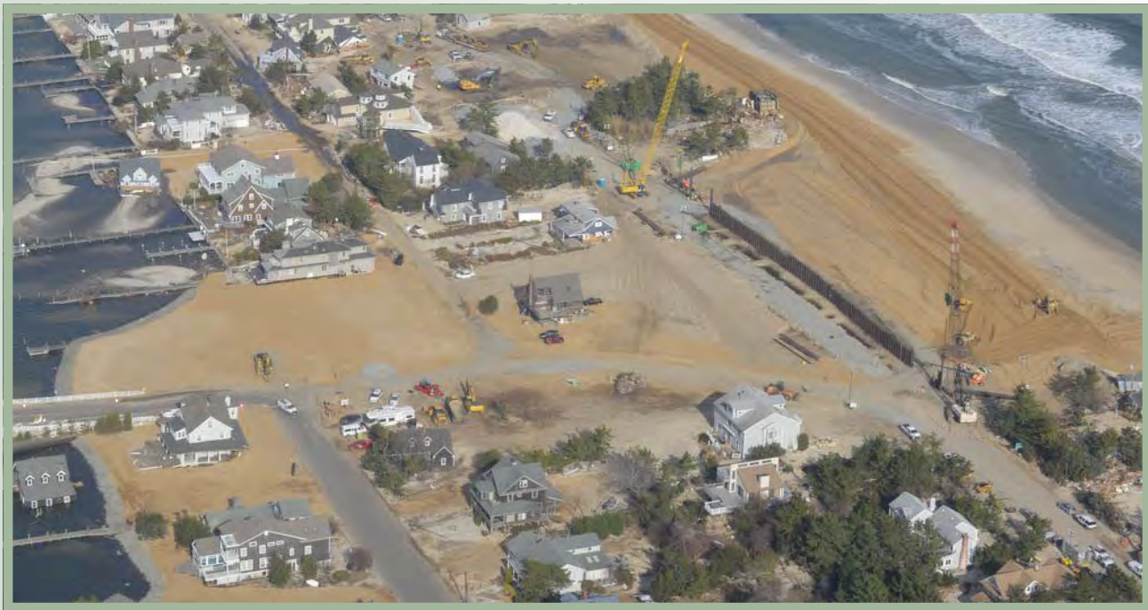
The Philadelphia District trucked in 86,000 tons of material to help fill the breach at Mantoloking, N.J.
