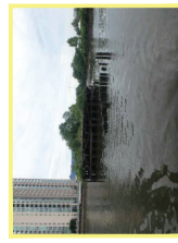
25 ISOLATED TIMBER PILES, VISIBLE DURING LOW TIDE
