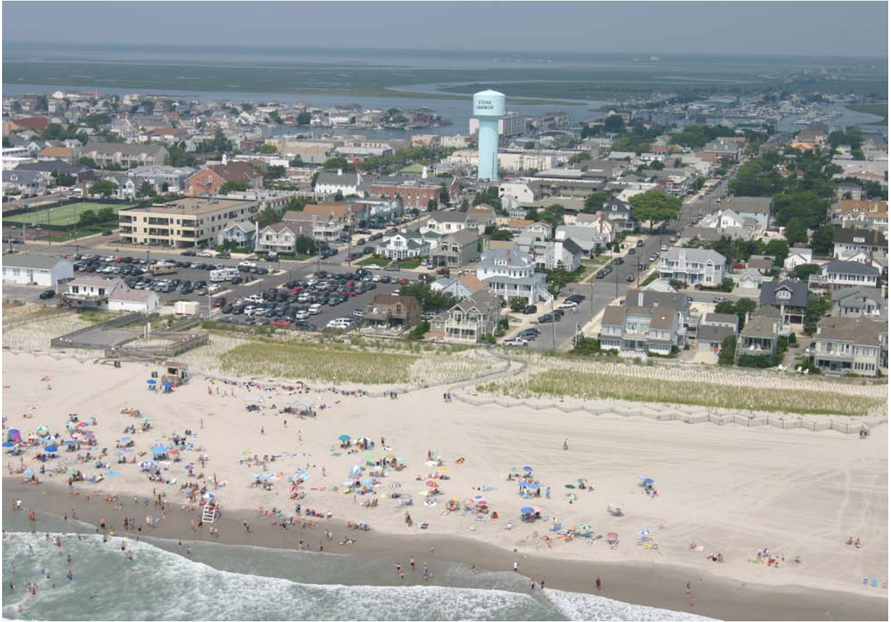
July 2004 after initial construction
