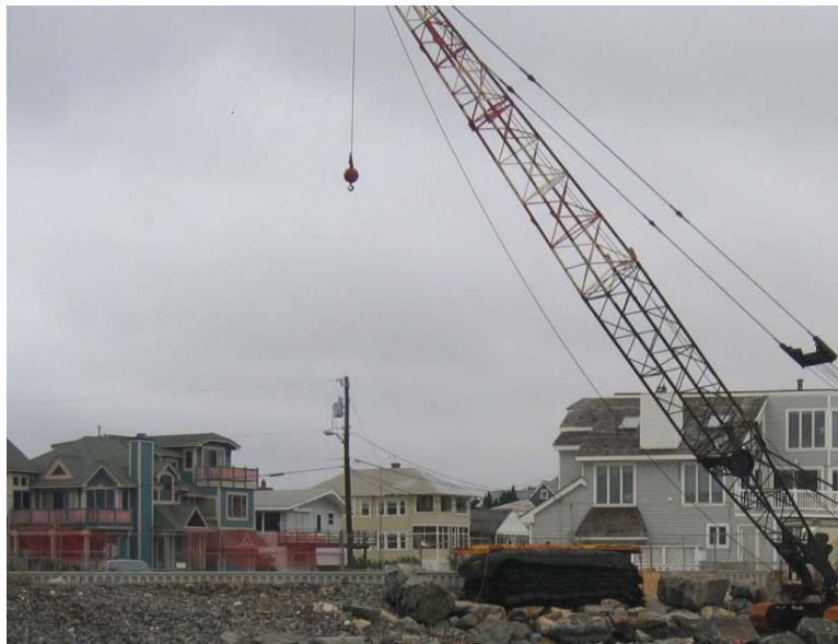
Hereford Seawall during construction
