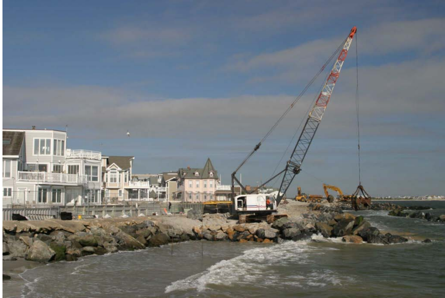
Avalon Seawall During construction
