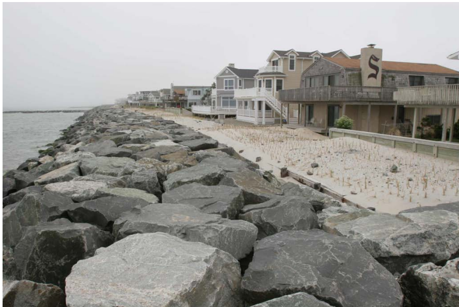
Avalon Seawall Completed Section
