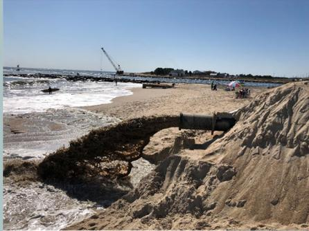
The state of Delaware operates the Indian River Inlet sand bypass plant in Sussex County, DE. Sand is pumped from the south side to the sand-starved north side. Federal construction funds are used to reimburse the
