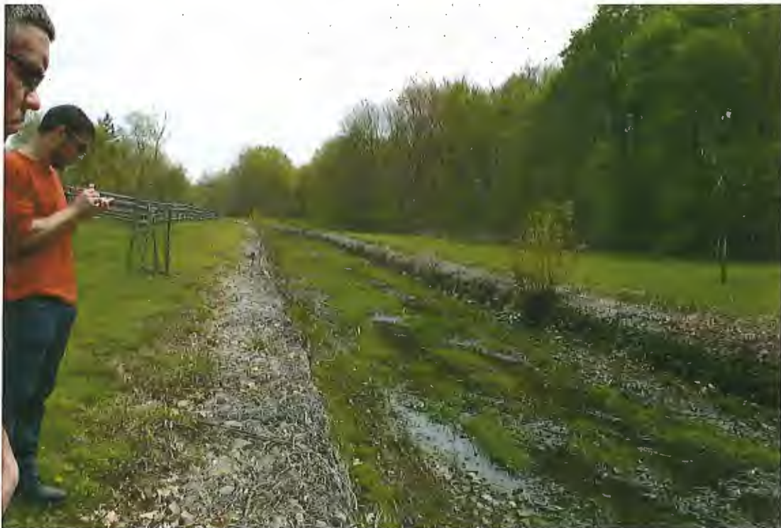
Figure 5: Gabion lined stream banks of Sandy Run Creek downstream of Figure 5 in Grove Park
