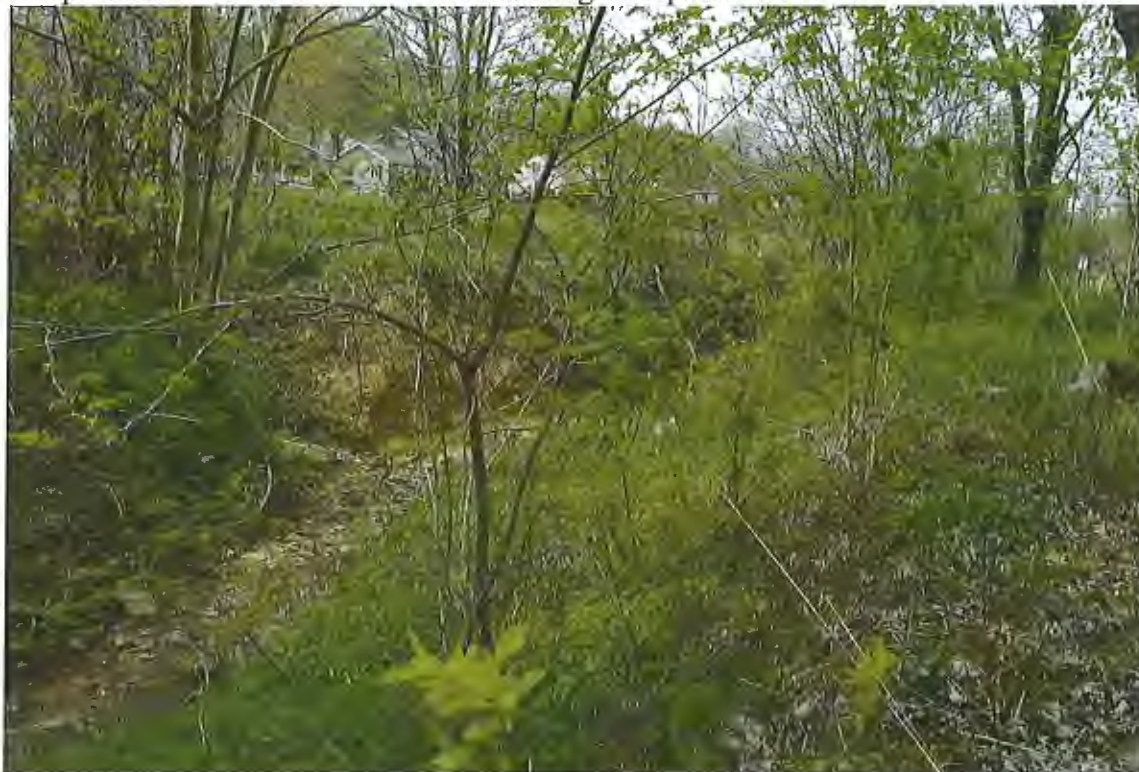
Figure 2: Eroded stream bank in Roychester Park
