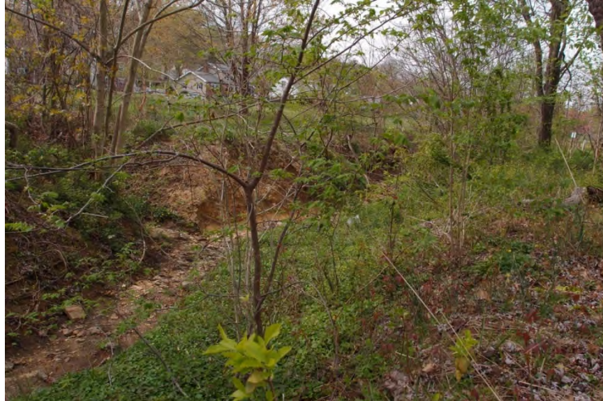
Figure 3: Eroded stream bank in Roychester Park
