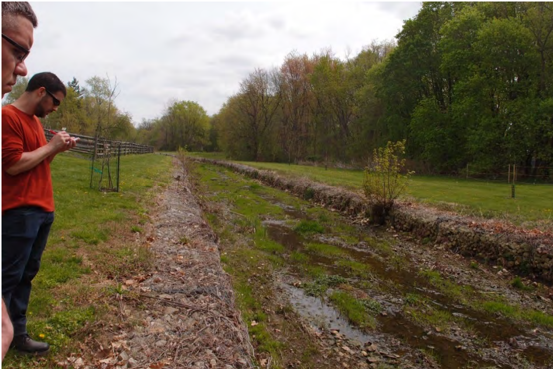
Figure 6: Gabion lined stream in Grove Park
