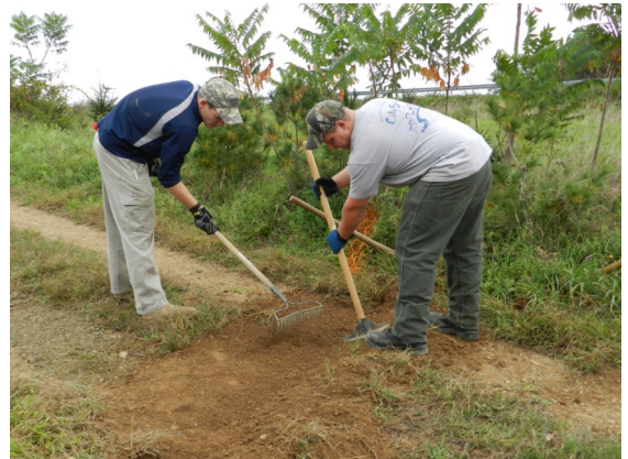
Kutztown University Volunteers Installing Water Bars Along the Hiking Trail
