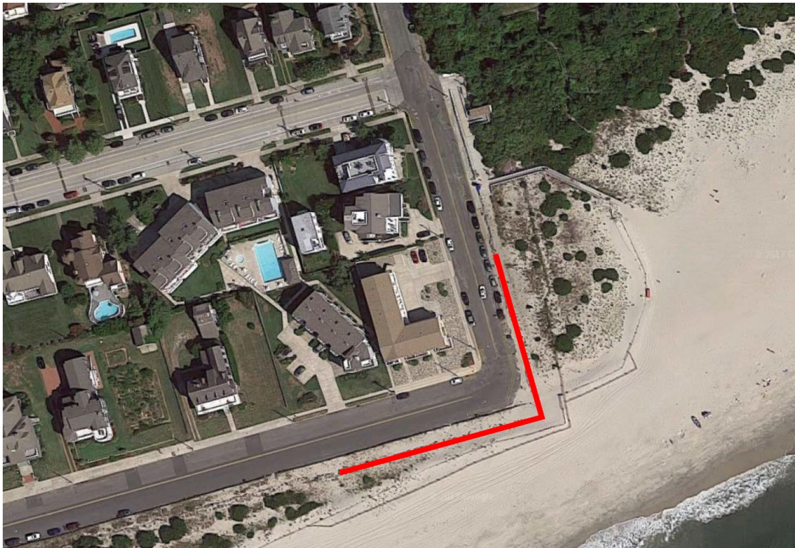
Area of seawall to be capped.
