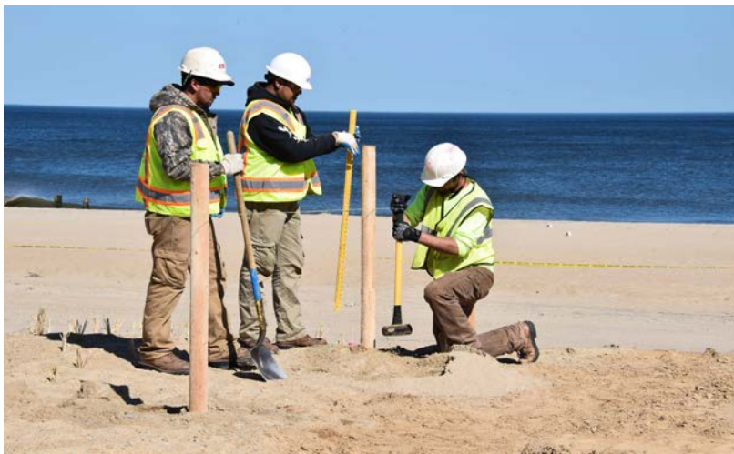
Left - a crew constructs fencing after beachfill operations were completed at Rehoboth Beach in 2016-2017.
