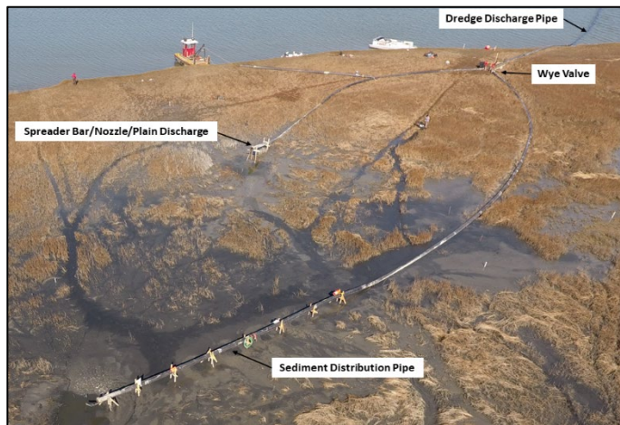
Little to no turbidity plume, outside of the tidal creek mouth on NE side of island.
