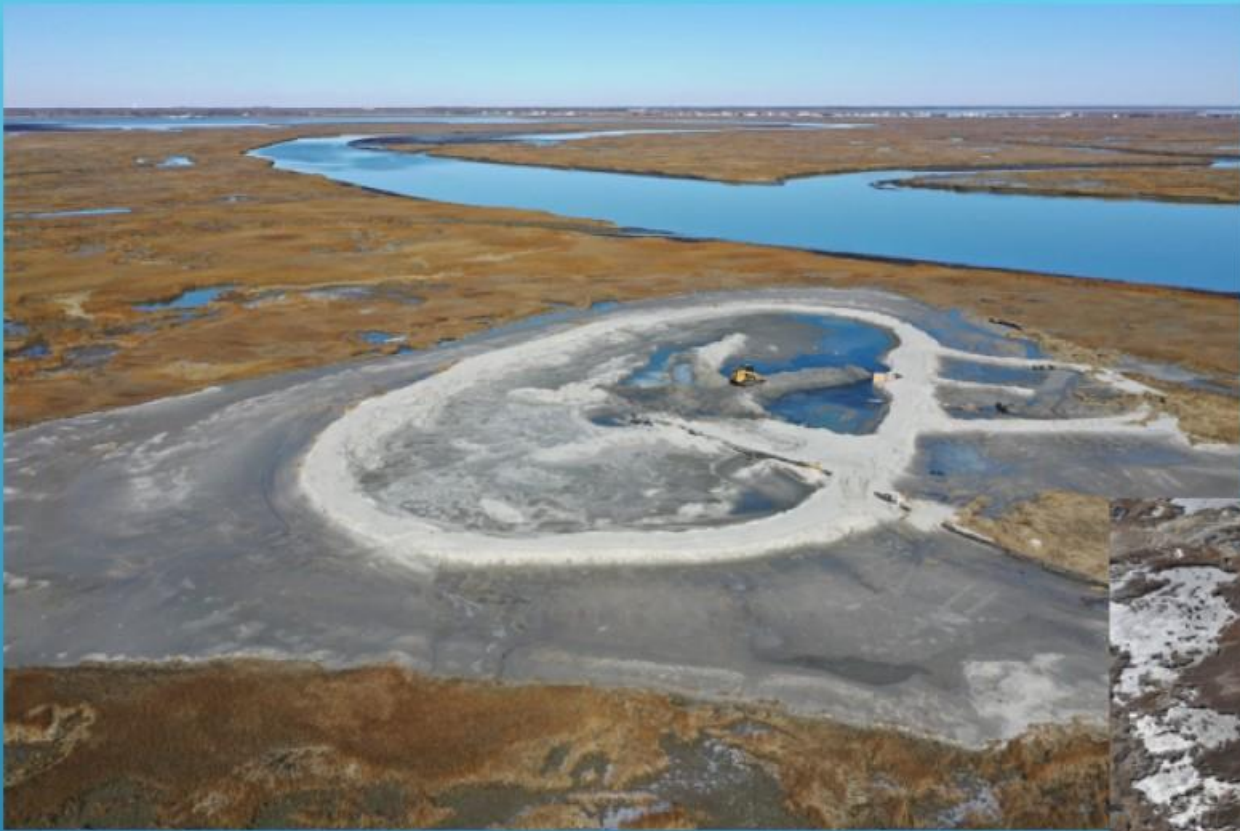
Phase One – Southern Cell Fill
