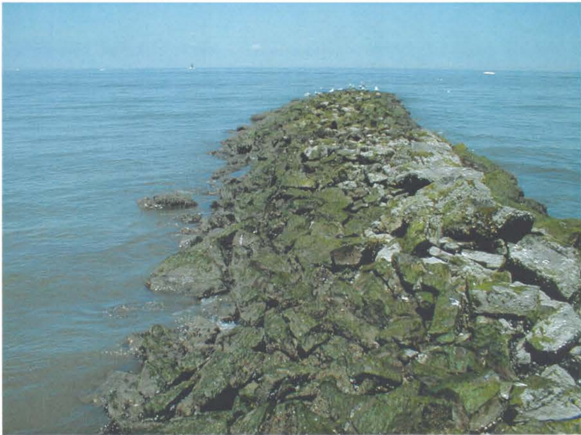
Figure 14. Old Inlet Jetty, 21 July 2001, 38° 48.743' N, 75° 11.668' W. Wide photograph from mid-jetty towards bay showing sandbuilder reef on flanks of jetty structure.
