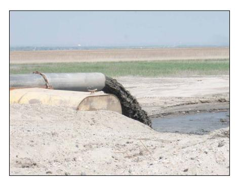
Figure 6-6. Dredged slurry being pumped into the Killcohook CDF during Reach C Deepening during the 2010 monitoring
