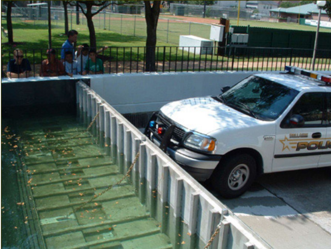
FloodBreak barrier in operation
