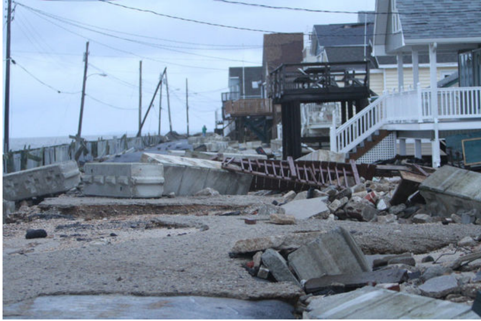
Photo 5: Damage following Hurricane Sandy in Gandys Beach
