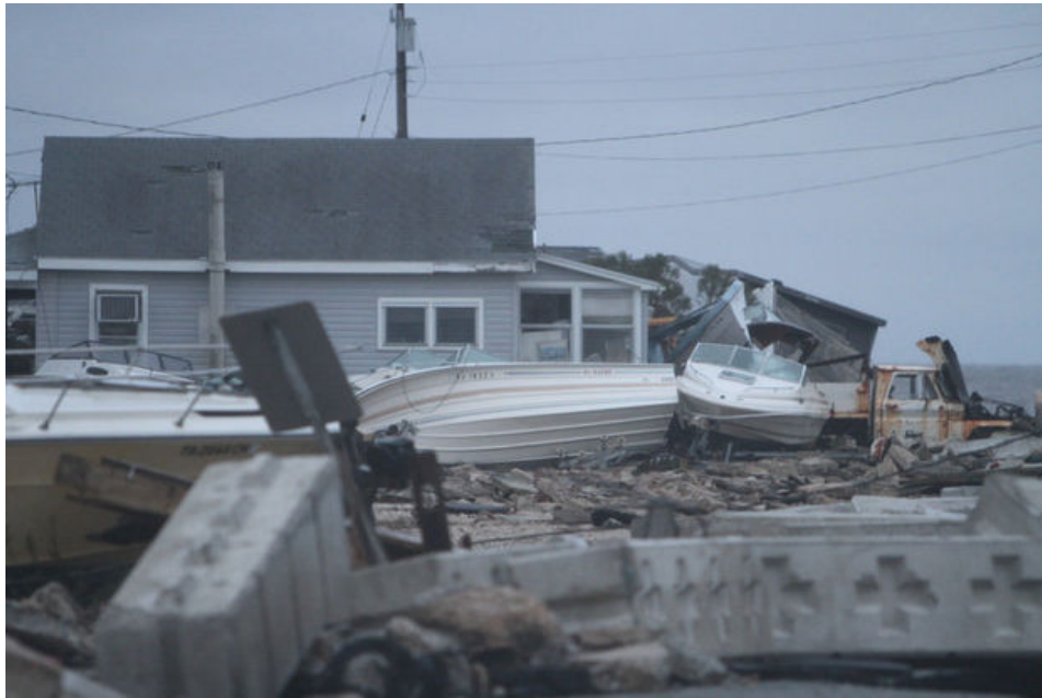
Photo 8: Damage following Hurricane Sandy in Gandys Beach
