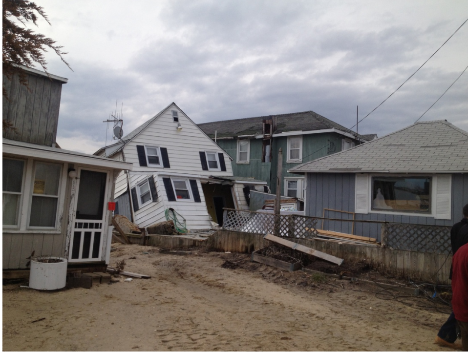
Photo 1: Damage following Hurricane Sandy in Fortescue
