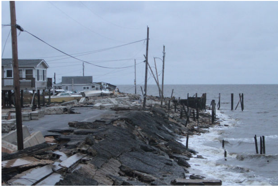
Photo 6: Damage following Hurricane Sandy in Gandys Beach
