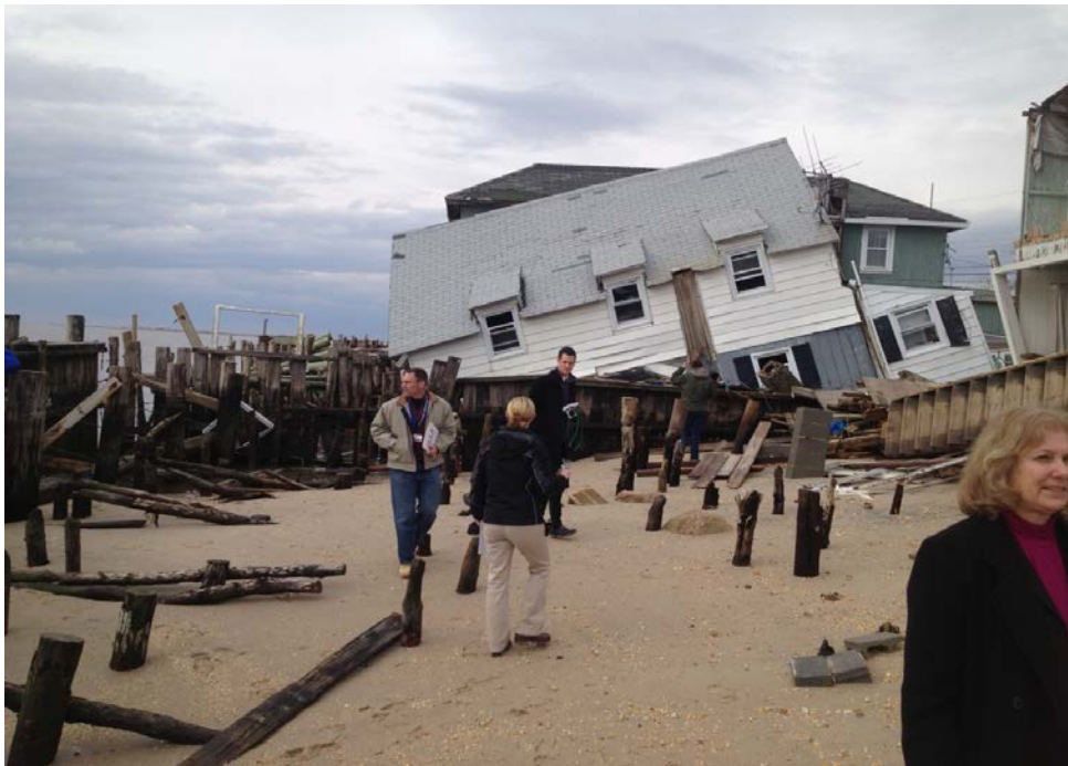
Photo 2: Damage following Hurricane Sandy in Fortescue
