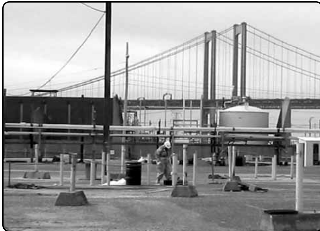
OU1 groundwater monitoring wells
