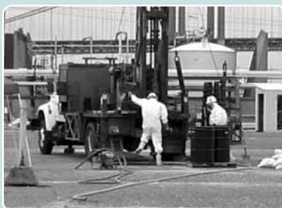
Monitoring well installation
