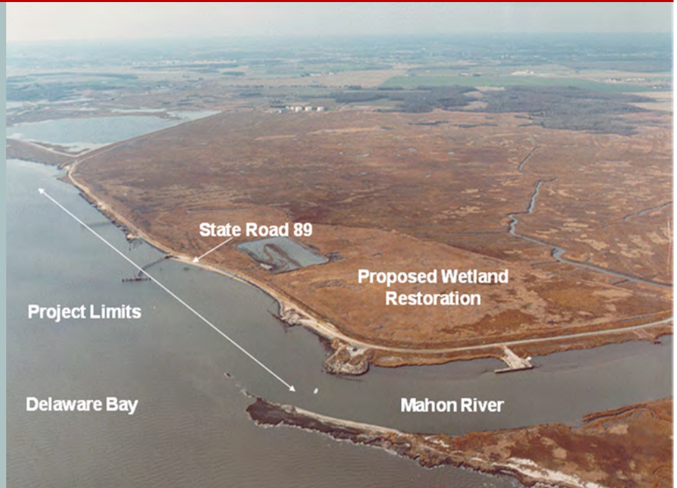
Overview of Project Site in Port Mahon, DE
