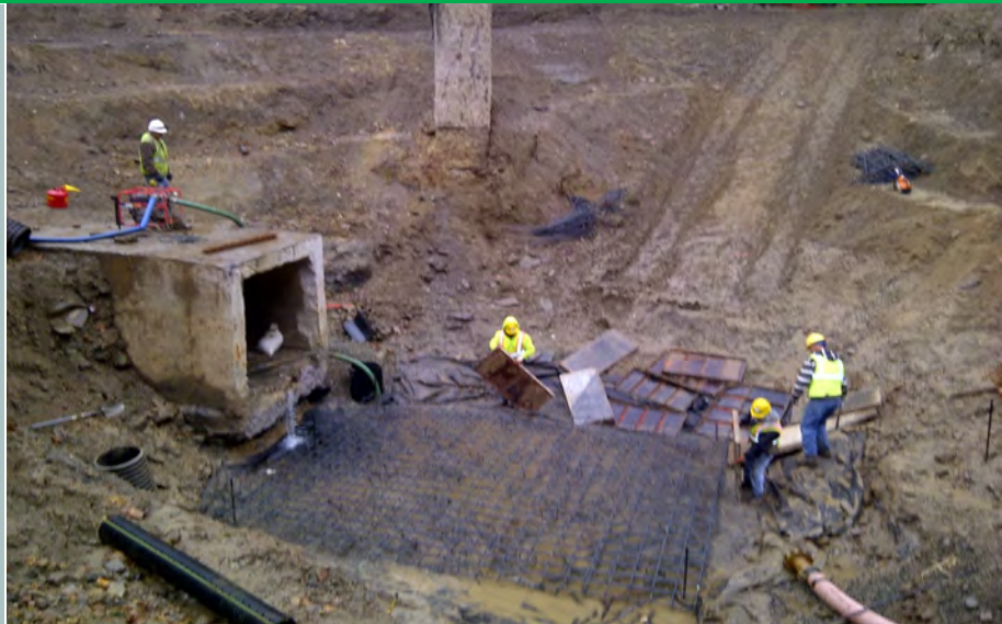
Construction of a vault structure to control sewer overflow, Philadelphia, PA
