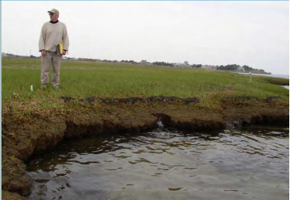
Erosion along the coastline.
