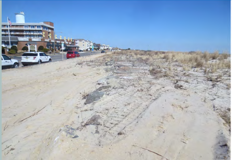
Existing seawall located along Beach Ave.
