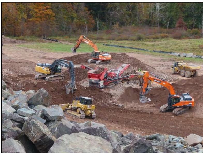
JADWIN DAM: The U.S. Army Corps of Engineers and its contractor constructed a Dam Safety Modification project at Jadwin Dam in Wayne County, PA. Work involved the installation of a geosynthetic liner system on part of the upstream slope and crest of the dam.
