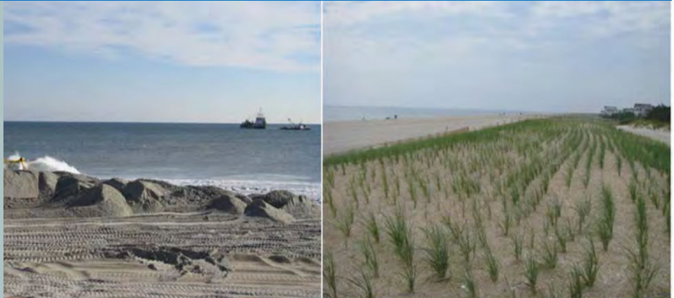
Preconstruction & During Construction
