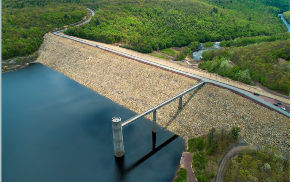
Aerial view showing Francis E. Walter Dam
