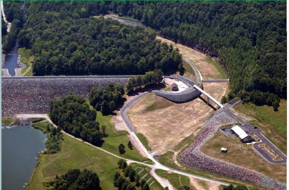
Aerial view showing Prompton Lake Dam
