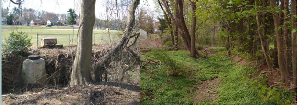
Left: Exposed manhole at Roychester Park Right: Historic channel at Grove Park
