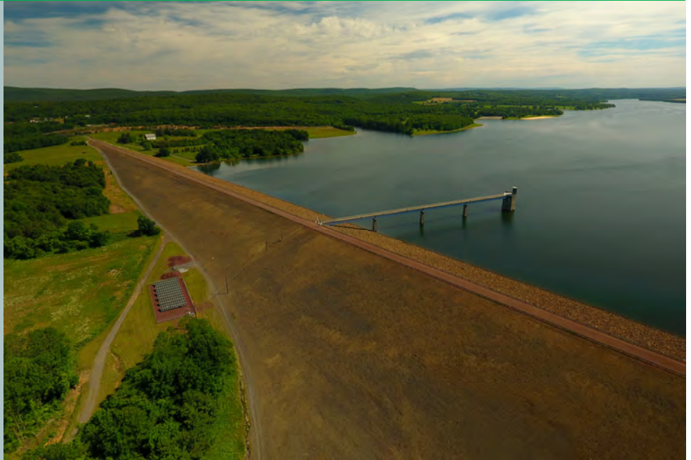
Aerial view of the earth and rock filled dam—Beltzville Lake, PA
