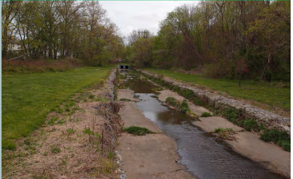
Existing concrete lined channel at Grove Park, Abington, PA
