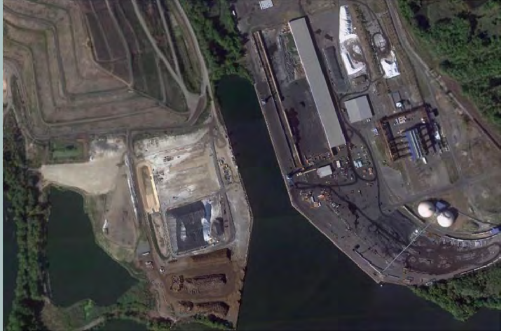
Port of Bucks County—Fairless Turning Basin
