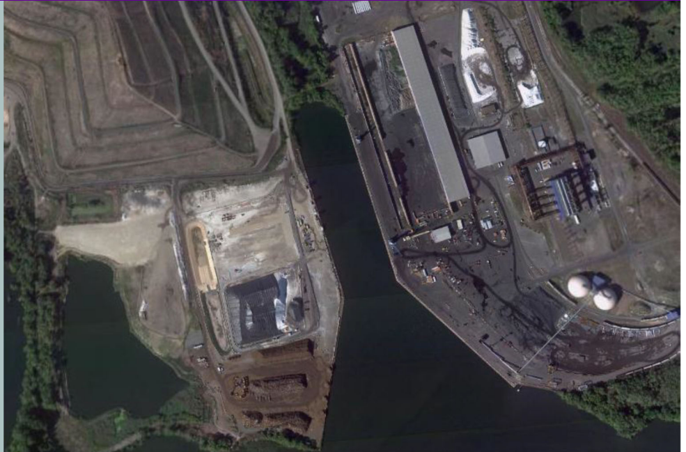
Port of Bucks County—Fairless Turning Basin
