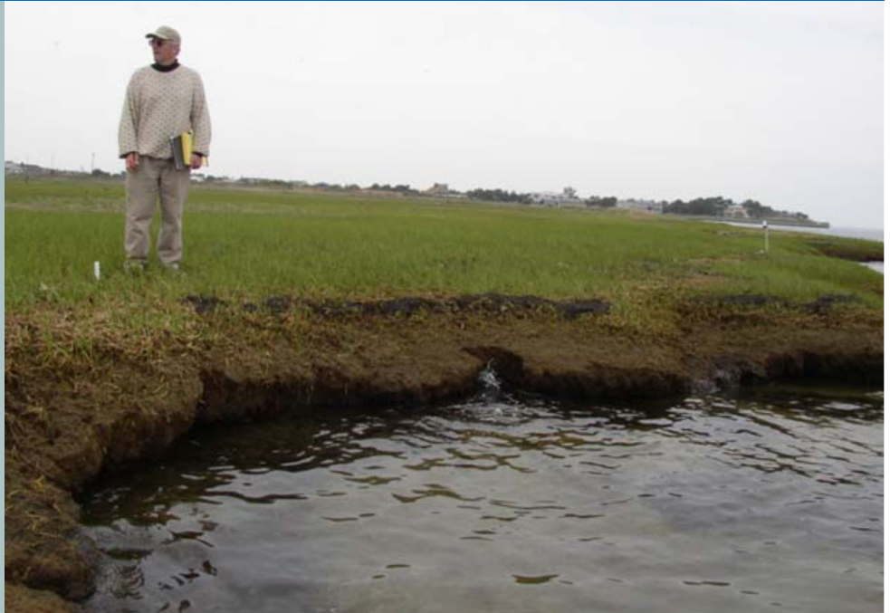
Erosion along the coastline.
