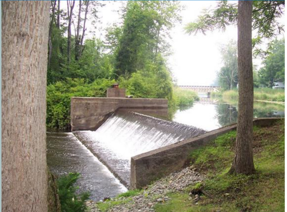
Tranquility Mill Dam, Pequest River, NJ
