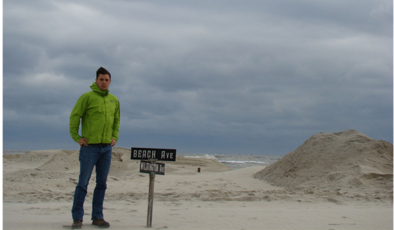
Approximately 6 feet of sand that was washed over the seawall and onto the street at the corner of Wilmington Ave and Beach Ave during Hurricane Sandy.
