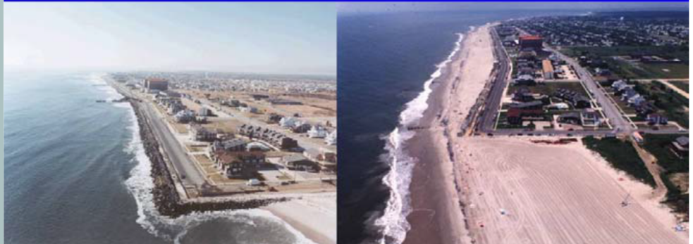
Aerial view of Initial Construction and Continued Periodic Nourishment, Cape May, NJ
