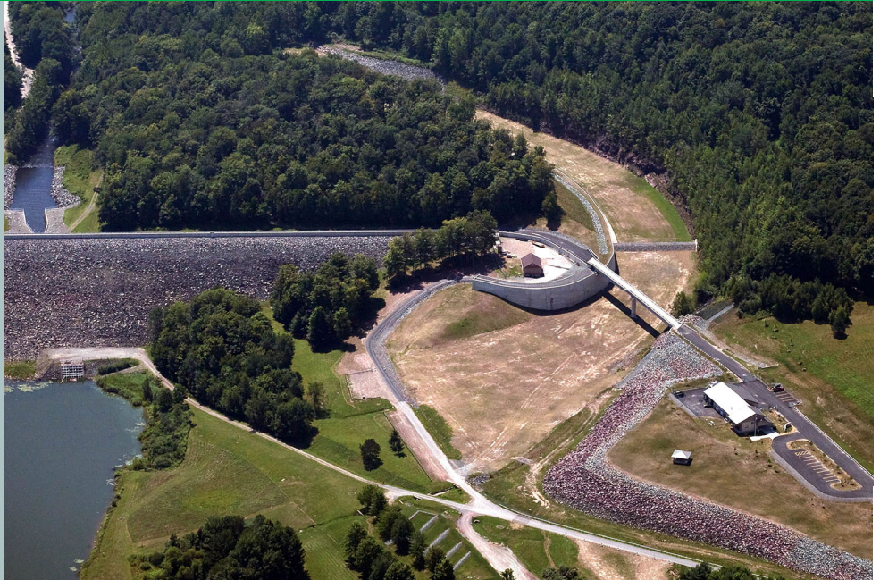
Aerial view showing Prompton Lake Dam
