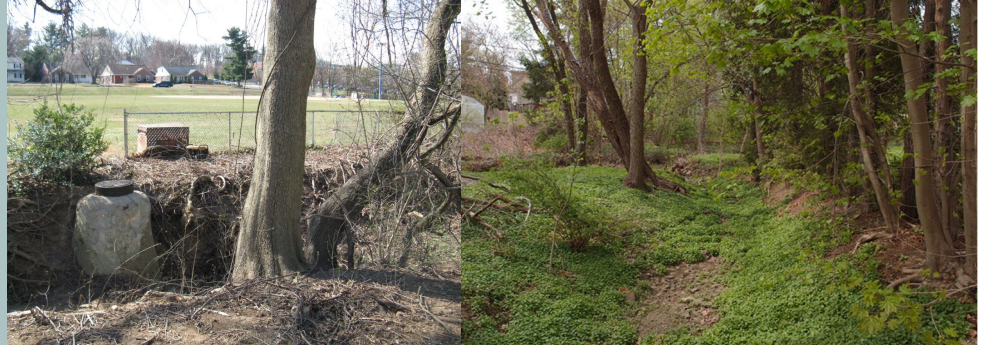
Left: Exposed manhole at Roychester Park Right: Historic channel at Grove Park
