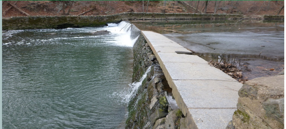
Roosevelt Boulevard Dam
