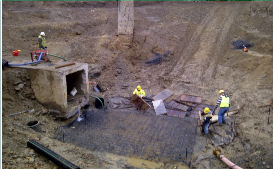
Construction of a vault structure to control sewer overflow, Philadelphia, PA
