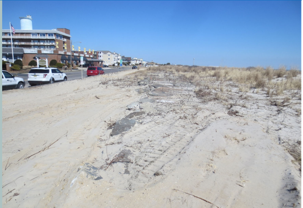
Existing seawall located along Beach Ave.
