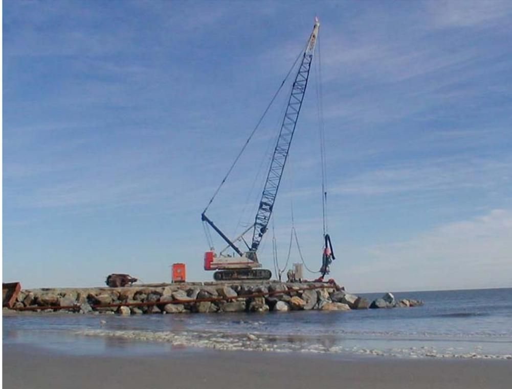
Figure 3. Crane deploying submersible pump from jetty
