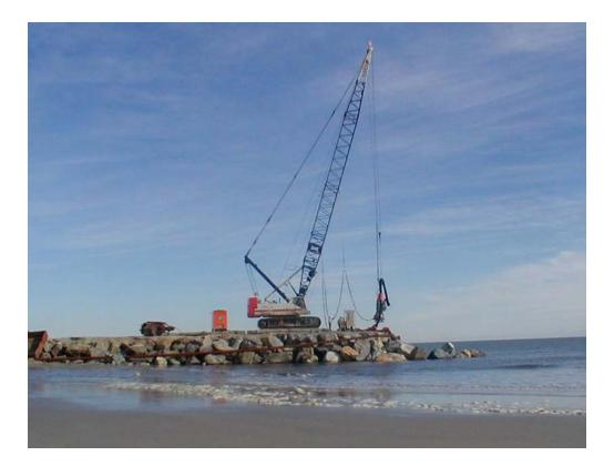
Figure 3. Crane deploying submersible pump from jetty
