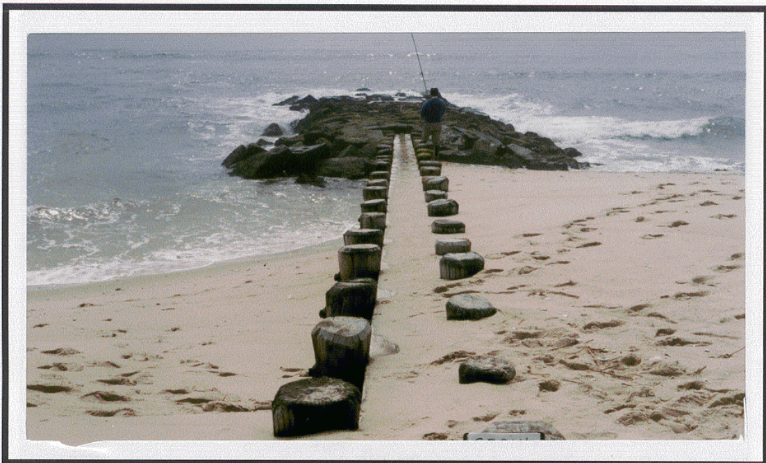
FIGURE 2-44 Typical Groin Configuration for LBI, Groin 38 at North 3rd Street Surf City
