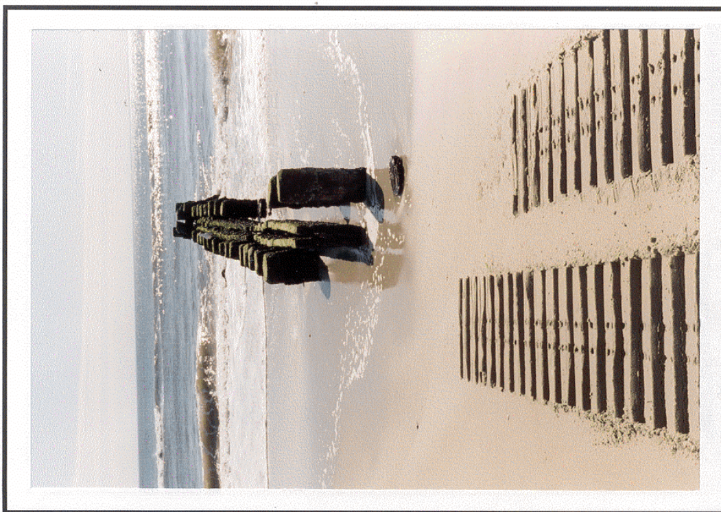
FIGURE 2-46 Example of Ineffective Notched Groin at 51st street, Brant Beach
