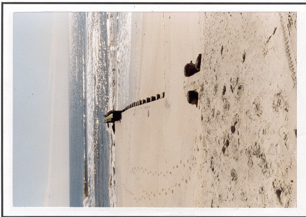
FIGURE 2-45 Effects of Notched Groin at 79th Street, Long Beach Township
