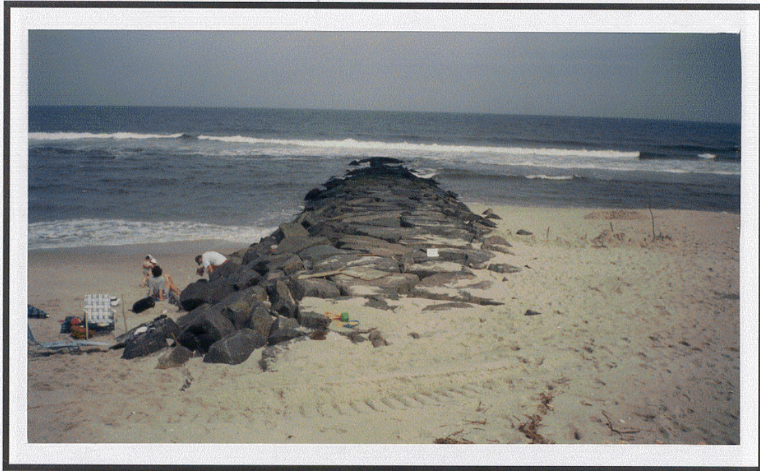
FIGURE 2-43 Groin 14 - Functional Stone Groin at 85th Street Harvey Cedars
