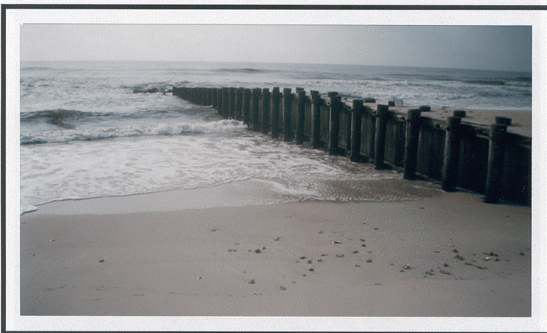
FIGURE 2-42 Groin 9, Low Permeability Timber Groin at Panorama So., (Loveladies) Long Beach Township
