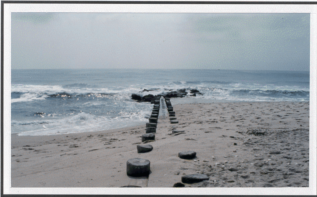
FIGURE 2-47 Combination Stone End and Low Profile Timber Groin at North Beach, Long Beach Township
