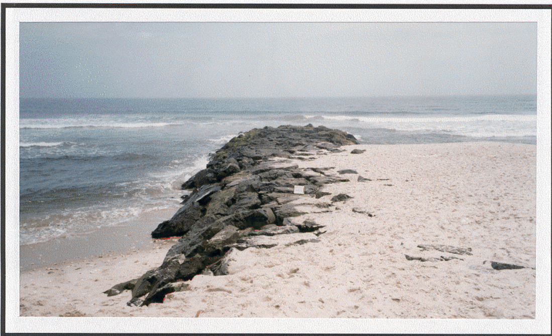
FIGURE 2-48 Higher Elevation all Stone Groin at 30th Street, Brant Beach, Long Beach Township
