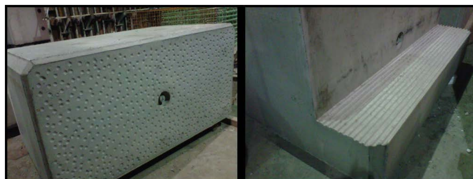
Examples of Textured Concrete. Source: USACE Buffalo District
