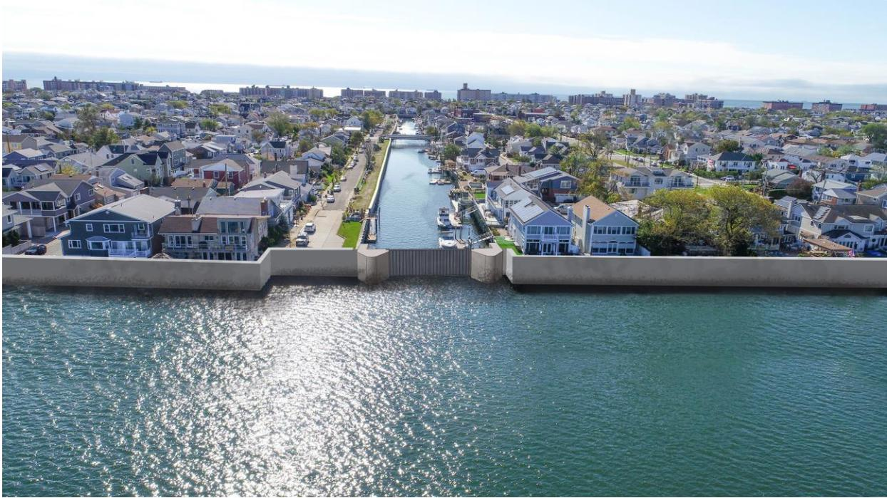
*Figure 39 - Rendering of Bayside View of Floodwall Around Long Beach*
