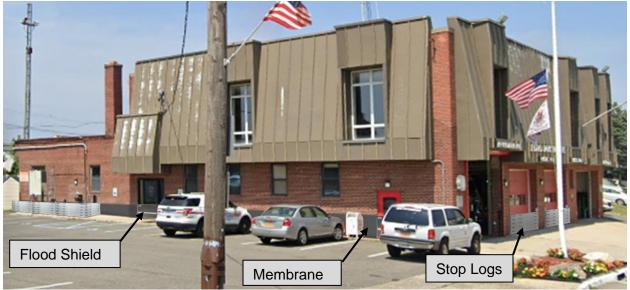
Figure 5.3.2 – Island Park FD Dry-Floodproofing Rendering (Courtesy of USACE-NAP)
