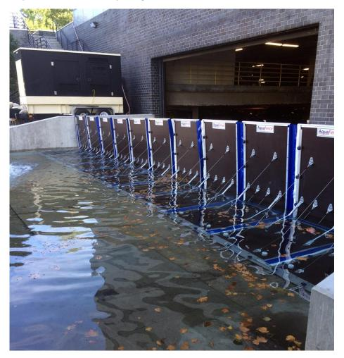
Figure 6.2.4 – AquaFence Non-Structural Measure in Use (Courtesy of Google Images)
