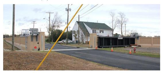
Figure 2.3.4.9 – Roller Gate Example – Port Monmouth, NJ (Courtesy of USACE-NAN)
