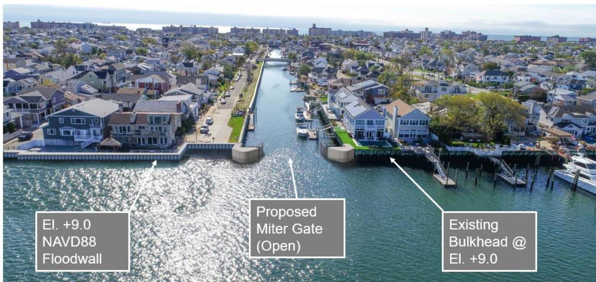
Figure 2.3.3.9 – NCBB Miter Gate – 20% AEP Plan (Courtesy of USACE-NAP)
