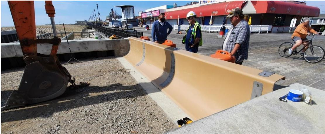
Figure 6.2.2 – Grant Avenue Fenceblade Barrier System (Courtesy of USACE-NAP)
