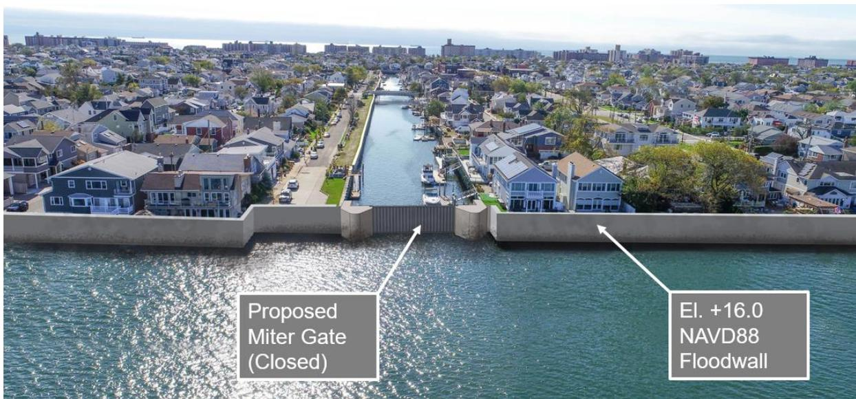
Figure 2.3.3.11 – NCBB Miter Gate – 1% AEP Plan (Courtesy of USACE-NAP)
