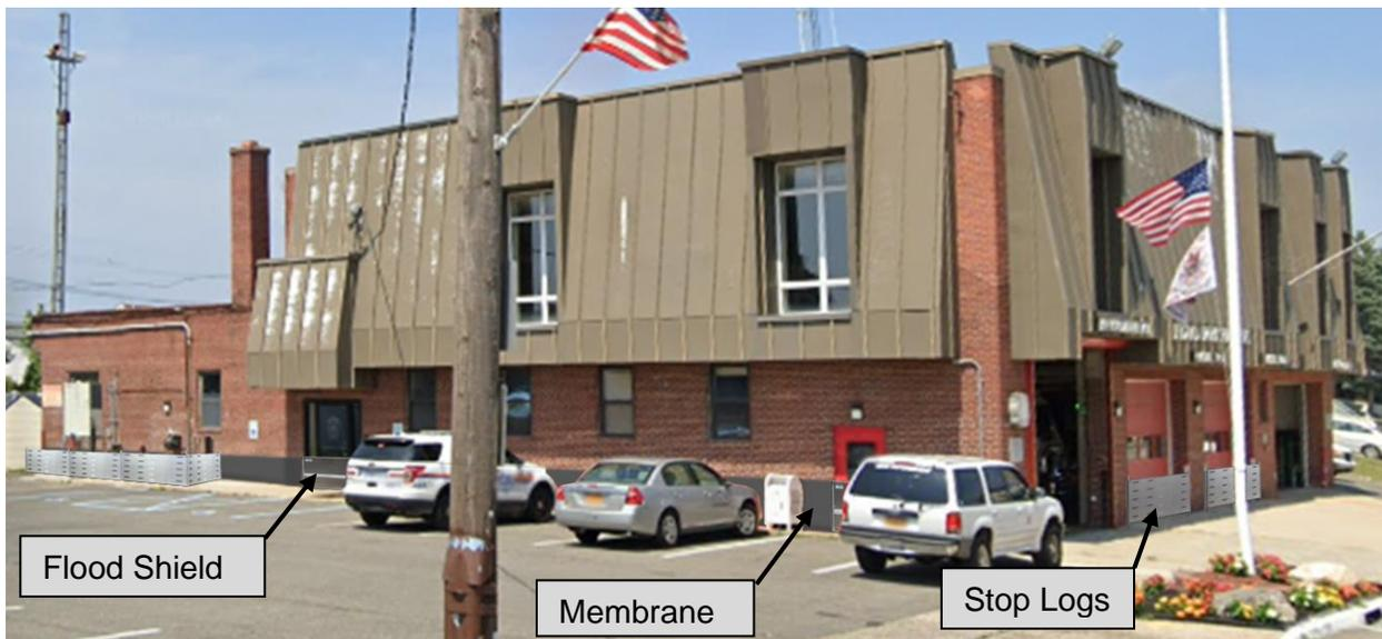
Figure 5.3.2 – Island Park FD Dry-Floodproofing Rendering (Courtesy of USACE-NAP)
