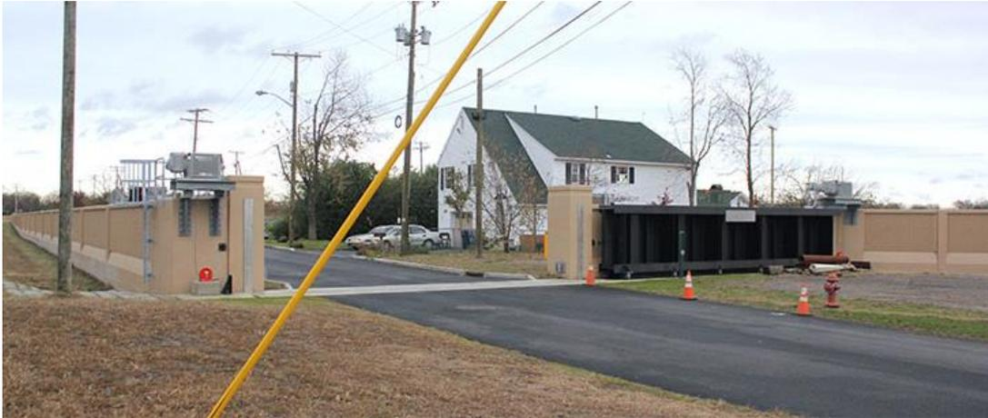
Figure 2.3.4.9 – Roller Gate Example – Port Monmouth, NJ (Courtesy of USACE-NAN)
