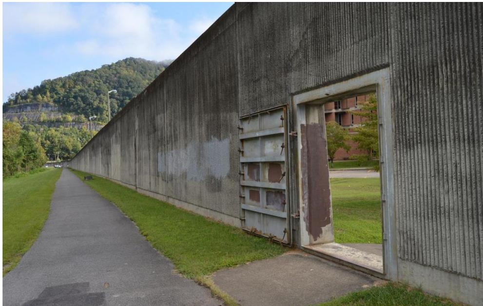
Figure 2.3.4.10 Swing Gate Example – Matewan, WV (Courtesy of USACE-LRH)
