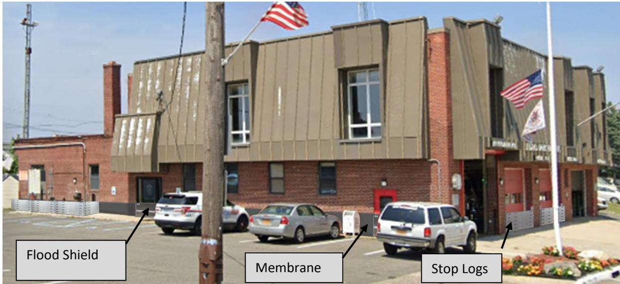
Figure 4 - Street View Example of Dry Flood Proofing
