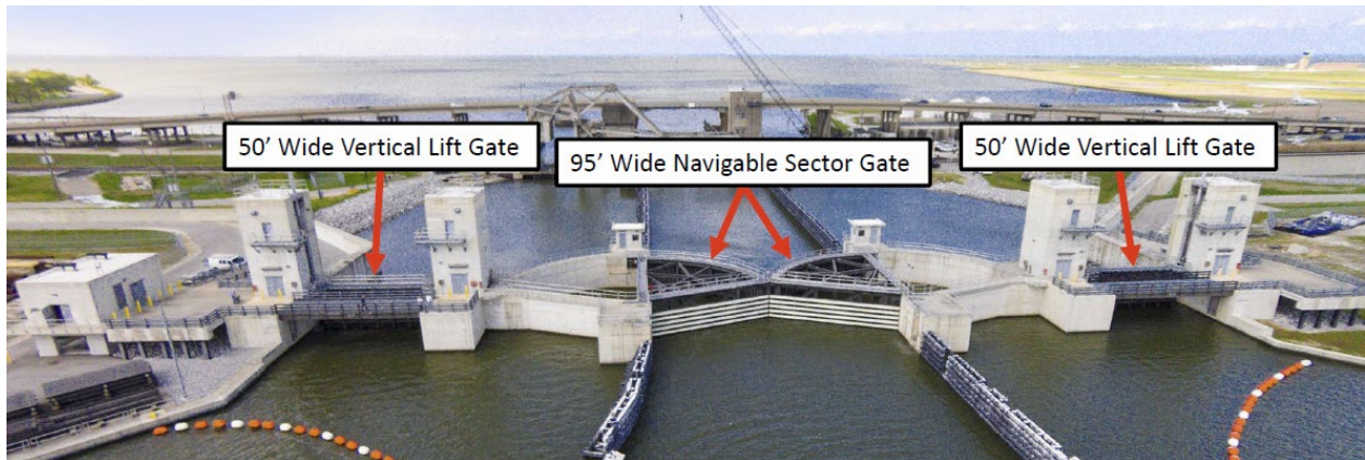
Figure 2: Seabrook Floodgate complex in New Orleans, LA.
