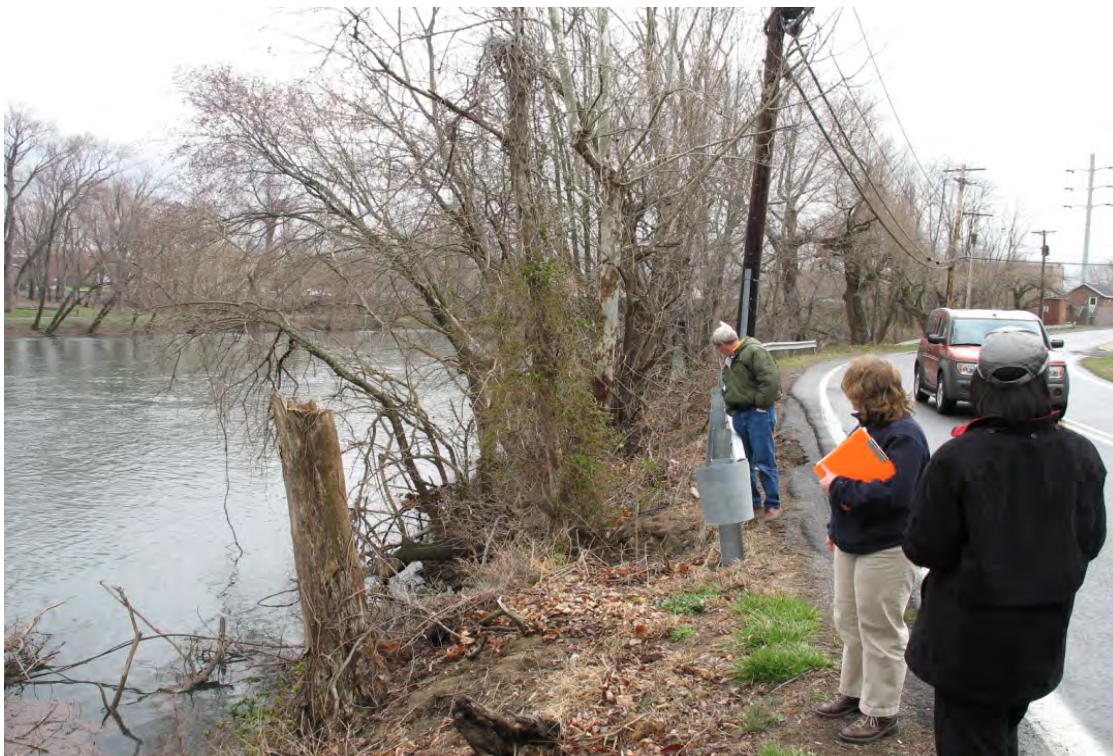
Figure 4. View of project area with the failing streambank (Photo 2008).
