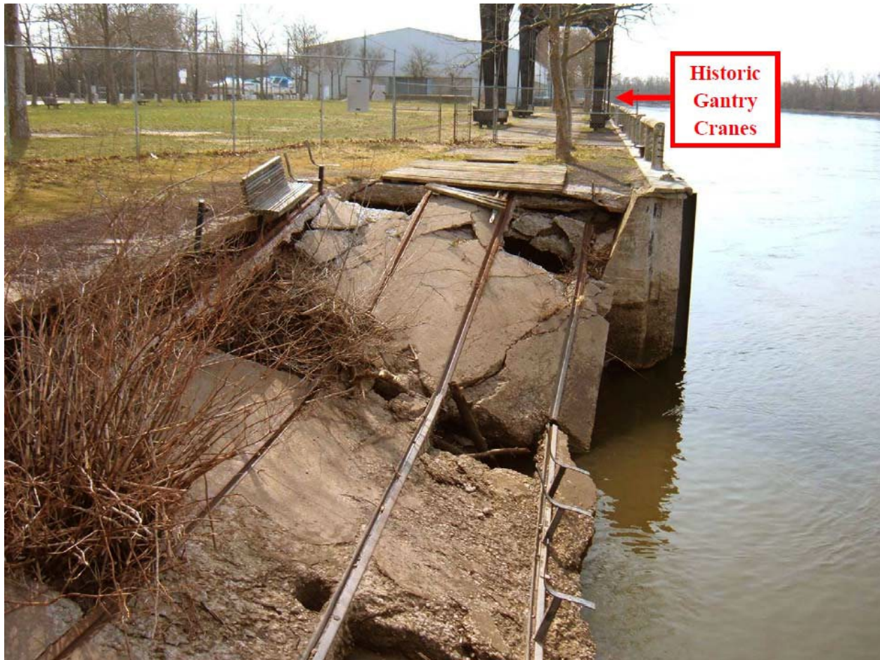
Figure 1-5: View of the project area looking south.
