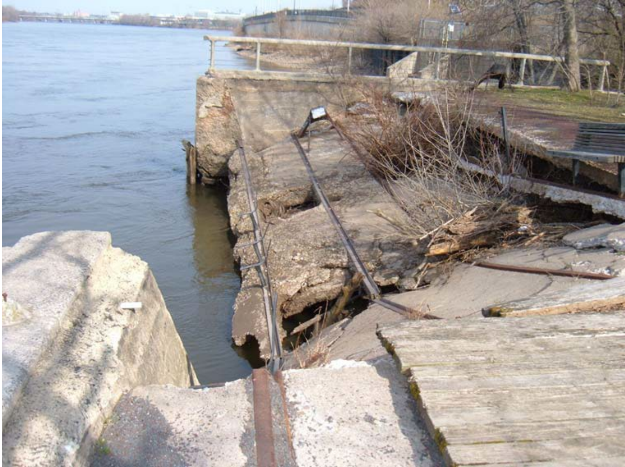
Figure 1-4: View of the project area looking north.
