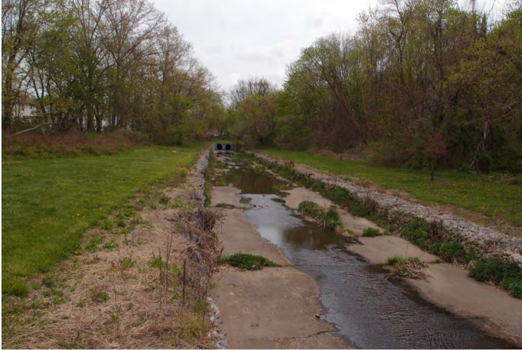
Figure 5: Concrete lined stream in Grove Park
