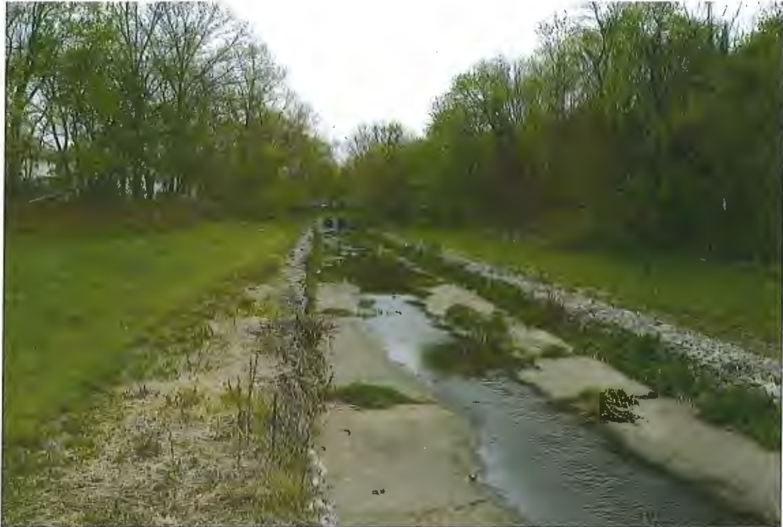
Figure 4: Concrete lined stream bottom with gabion baskets lining the stream banks of Sandy Run Creek in Grove Park
