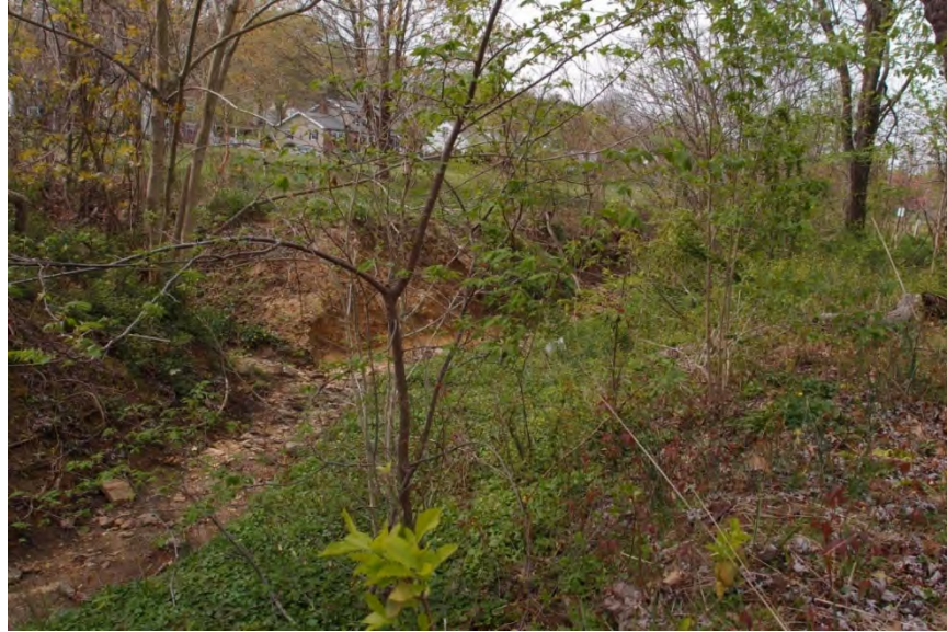
Figure 3: Eroded stream bank in Roychester Park
