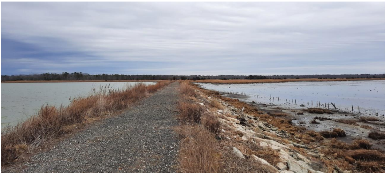
Figure 5: Heislerville dike looking east from the cross-dike junction, stable dike area (photo courtesy of J. Benigno, USACE).
