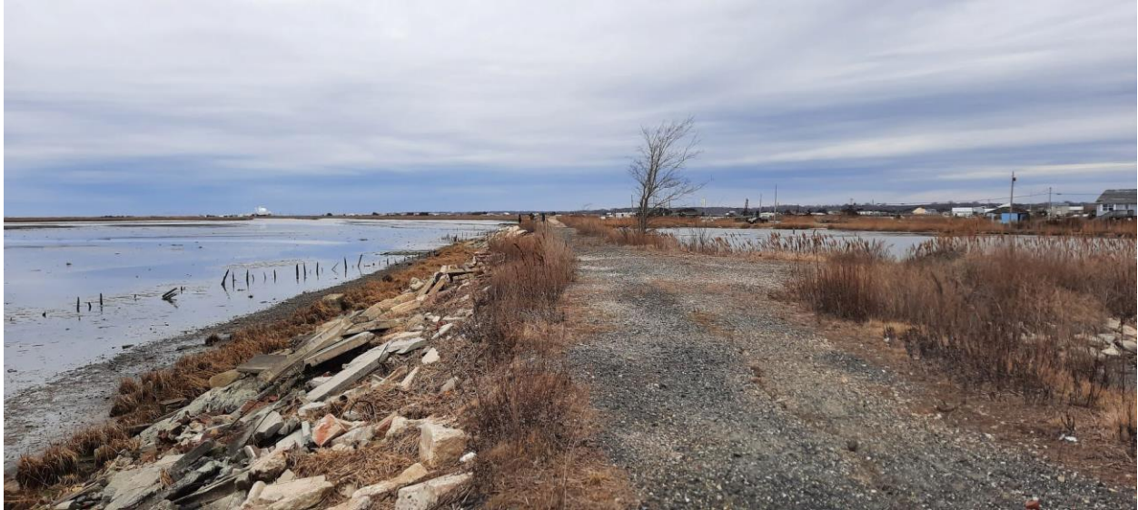
Figure 6: Heislerville dike looking west from the cross-dike junction: critical area of the Heislerville dike (photo courtesy of J. Benigno, USACE).
