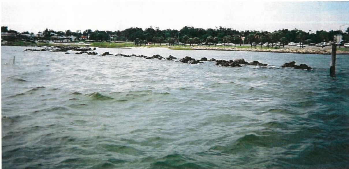
Figure 3. Visual comparison of the wave conditions seaward and landward of the structure.
