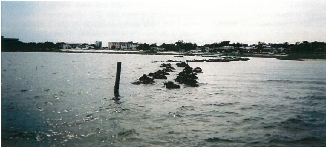
Figure 4. Wave propagation through the gap between the structure and the seawall (below the bottom of the picture). Note the reflected waves propagating nearly parallel to the structure.
