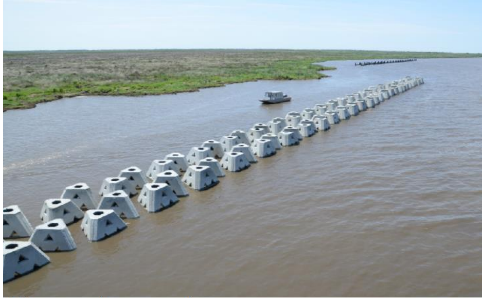
Figure A2-2: Wave Attenuation Devices (WADs) at Shark Island in New Iberia, LA
