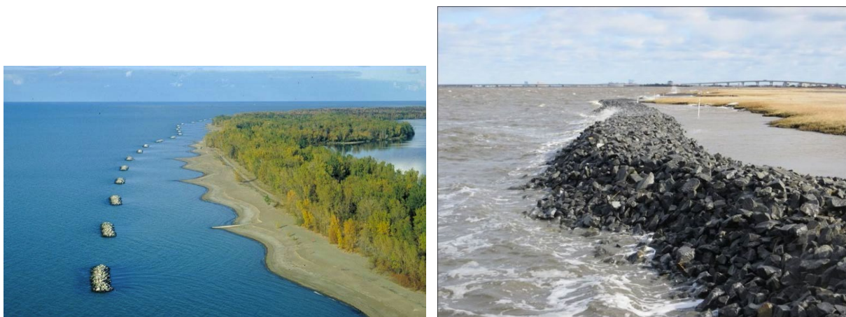
Figure 5.15: Stone Breakwaters
