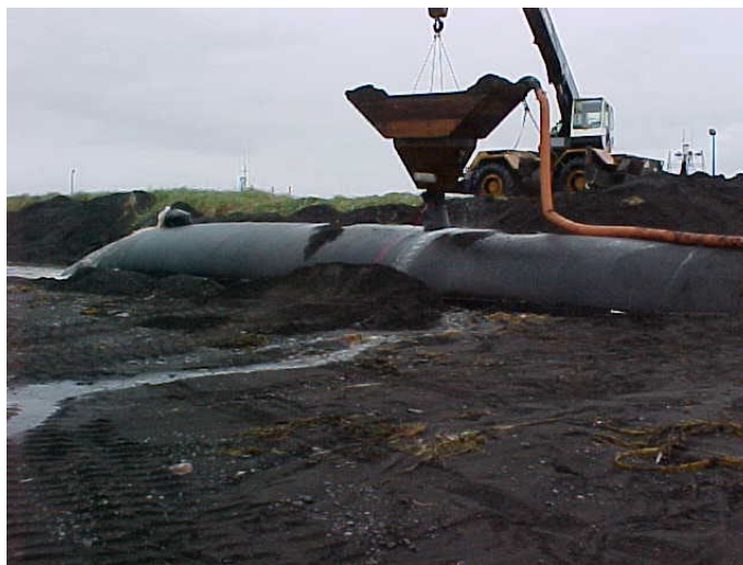
Figure 5.13: Corps Installation of Geotubes® at Nelson Lagoon, Alaska
