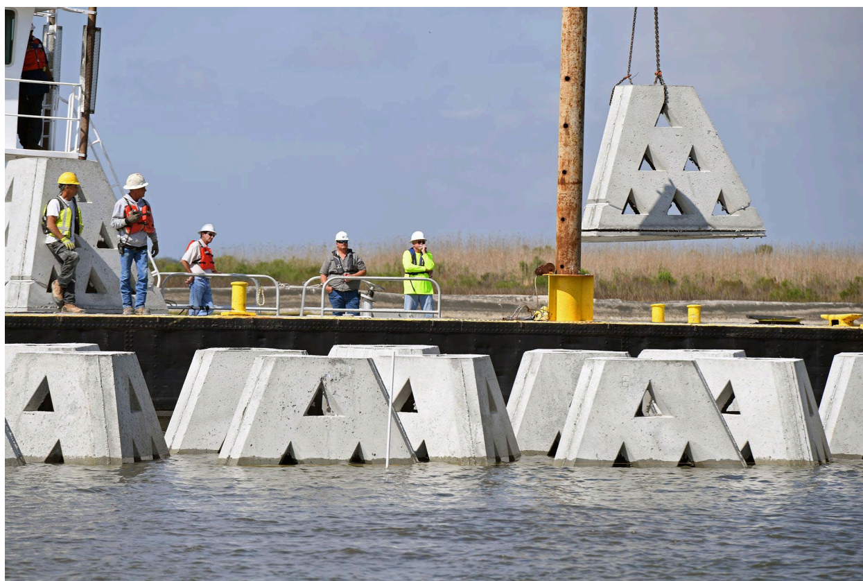
Figure 5.18: WADs® Placement at Bayou Caddy in Biloxi, MS
