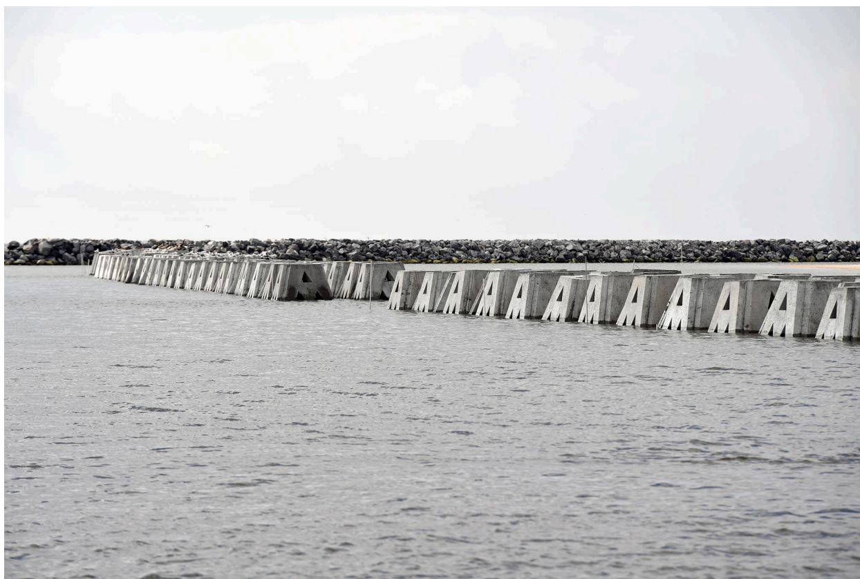
Figure 5.19: WADs® in Place at Bayou Caddy in Biloxi, MS
