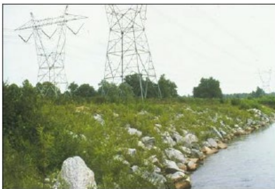
Figure 5.5: Stone Revetment with Planting
