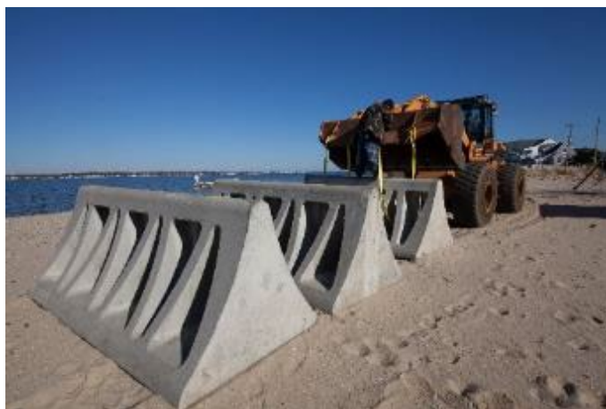
Figure 5.17: Beach Prisms™ Prior to Installation
