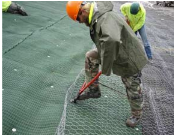
Figure 5.3: Installation of Turf Reinforcement Mat
