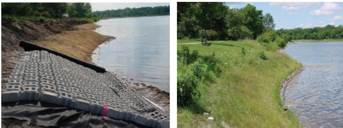
Figure 5.7: Articulated Concrete Mat Installation and Planted
