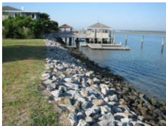
Figure 5.6: Stone Revetments
