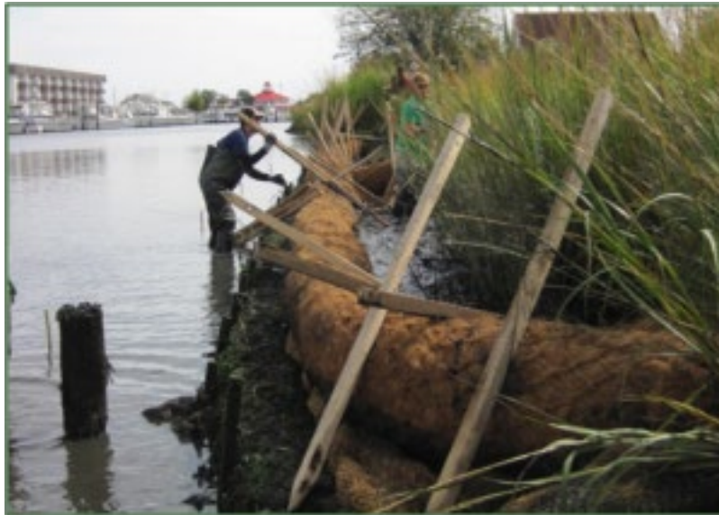
Figure 5.8: Installation of Biologs
