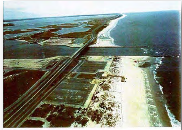
Figure 90. Indian River Inlet, Delaware fixed bypassing system (Photo courtesy of Tony Pratt, DNREC).
