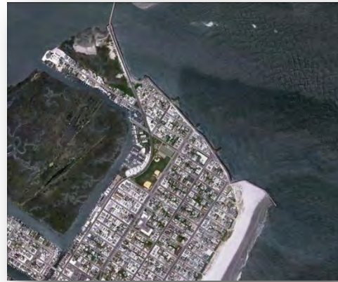
Figure 13. Erosion control structures along inlet frontage in Avalon.
