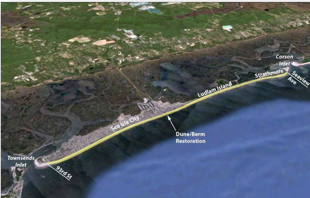
Figure 115. Great Egg Harbor to Townsends Inlet Authorized Shore Protection Project at Ludlam Island.
