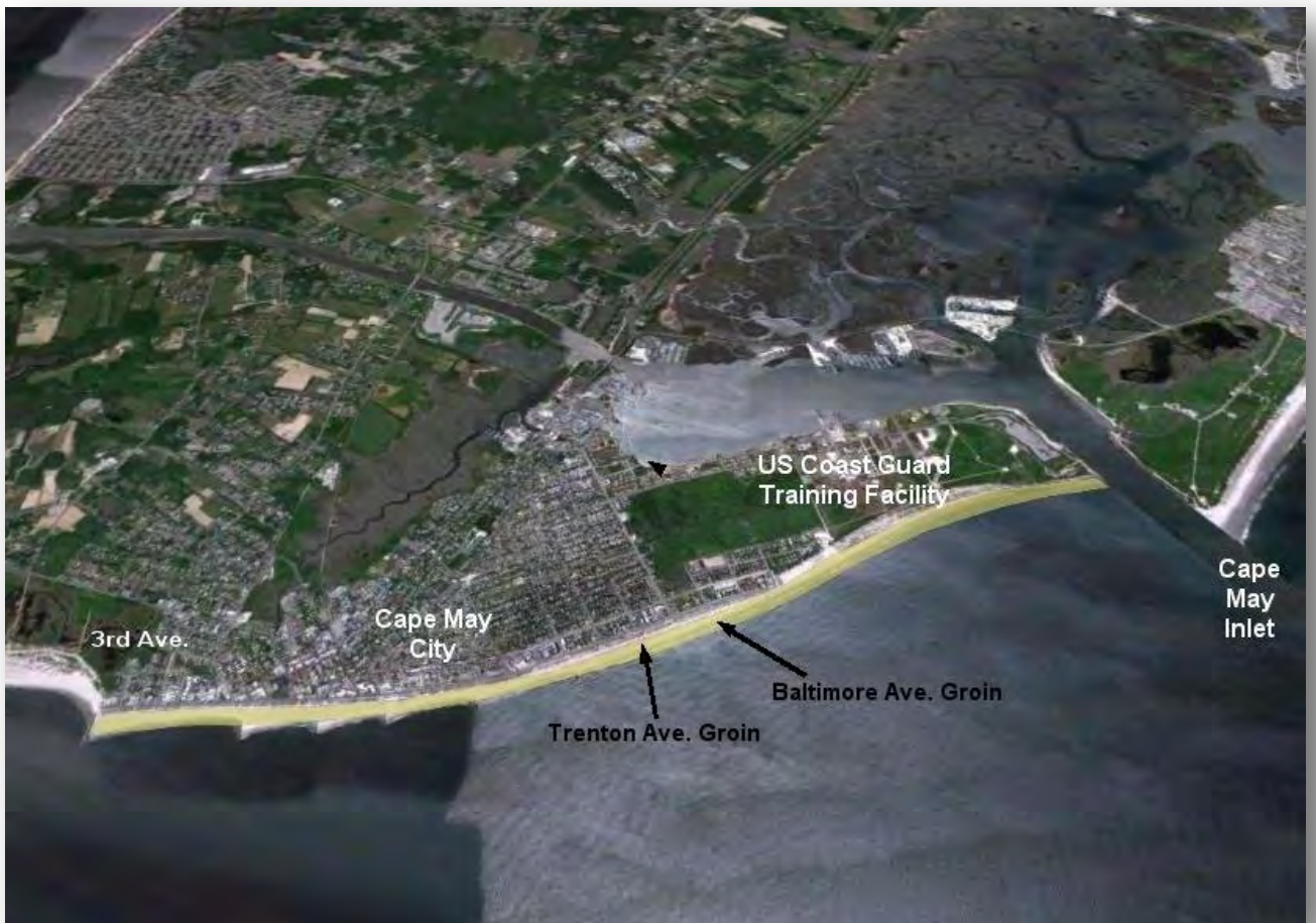
Figure 83. Cape May City Authorized Shore Protection Project.
