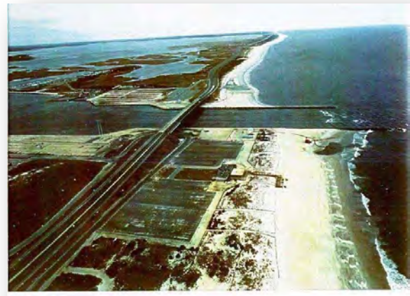
Figure 120. Indian River Inlet, Delaware fixed bypassing system (Photo courtesy of Tony Pratt, DNREC).
