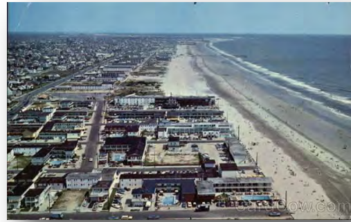
Figure 12. Development along Five Mile Beach in Wildwood Crest.
