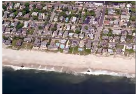
Figure 23. Groins in Bay Head.
