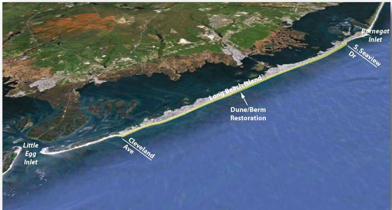
Figure 155. Barnegat Inlet to Little Egg Inlet (Long Beach Island) Authorized Shore Protection Project.
