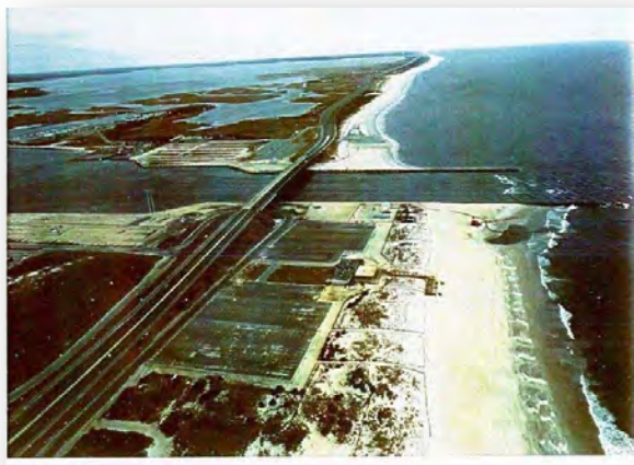
Figure 171. Indian River Inlet, Delaware fixed bypassing system (Photo courtesy of Tony Pratt, DNREC).
