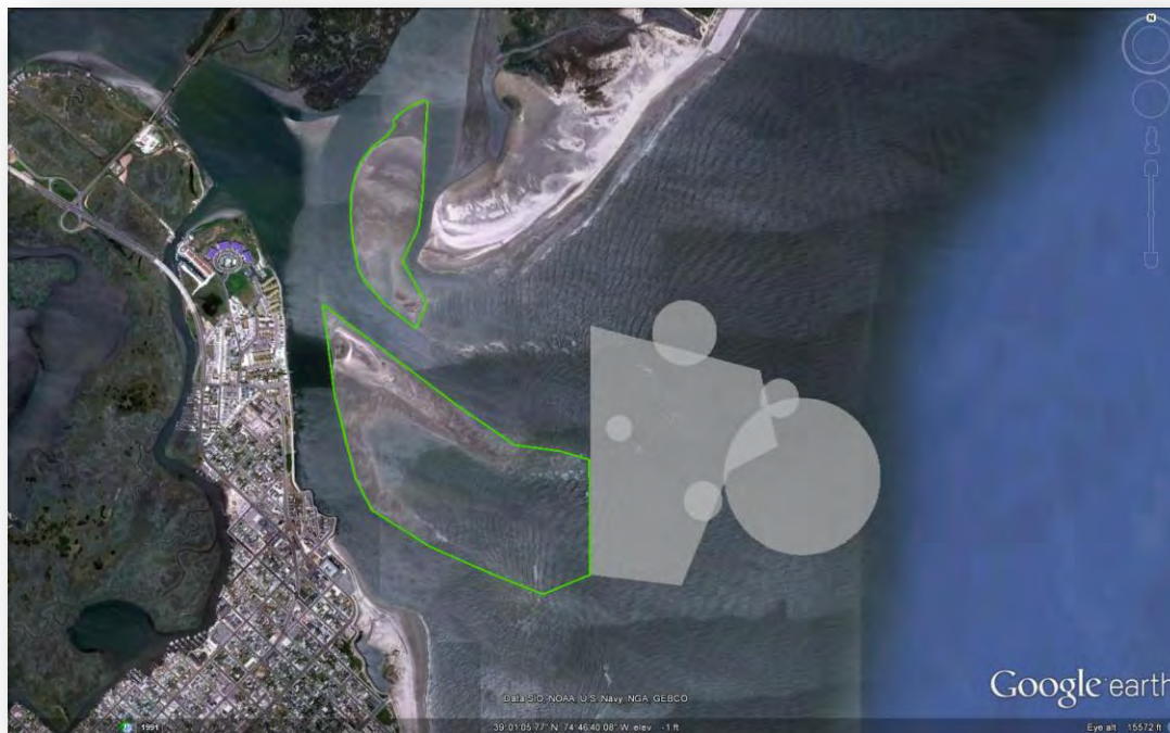
Figure 104. Potential borrow areas (green) at the ebb and flood tidal shoals of Hereford Inlet. Permitted borrow areas shown as shaded white. Image courtesy of Google Earth®.
