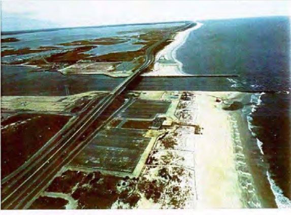
Figure 160. Indian River Inlet, Delaware fixed bypassing system (Photo courtesy of Tony Pratt, DNREC).
