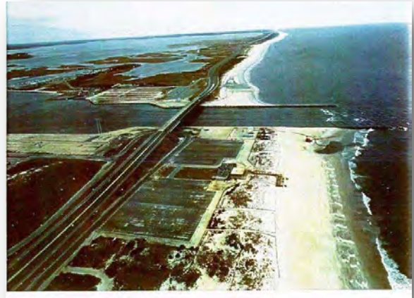
Figure 183. Indian River Inlet, Delaware fixed bypassing system (Photo courtesy of Tony Pratt, DNREC).
