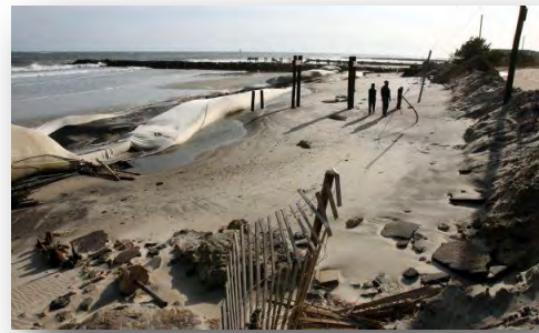
Figure 16. 2009 storm damage to Ocean City geotextile sand bags.
