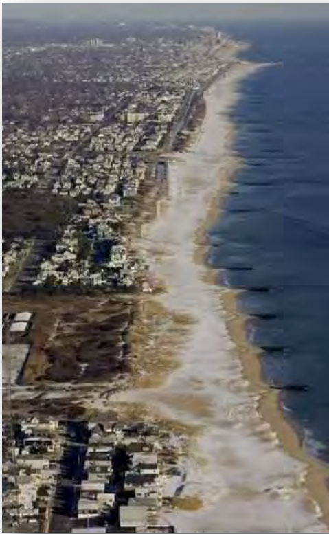
Figure 25. Groin field north of Manasquan Inlet.
