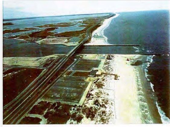
Figure 143. Indian River Inlet, Delaware fixed bypassing system (Photo courtesy of Tony Pratt, DNREC).
