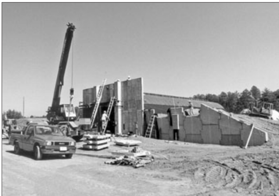
Fort Dix ammunition storage facility under construction
