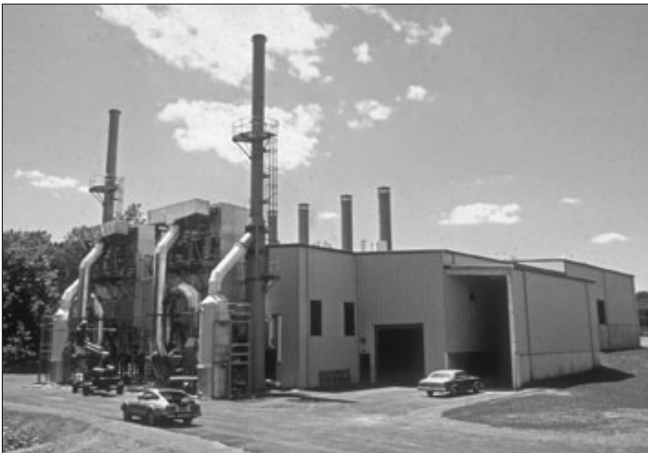
Resource Recovery Facility, Fort Dix
