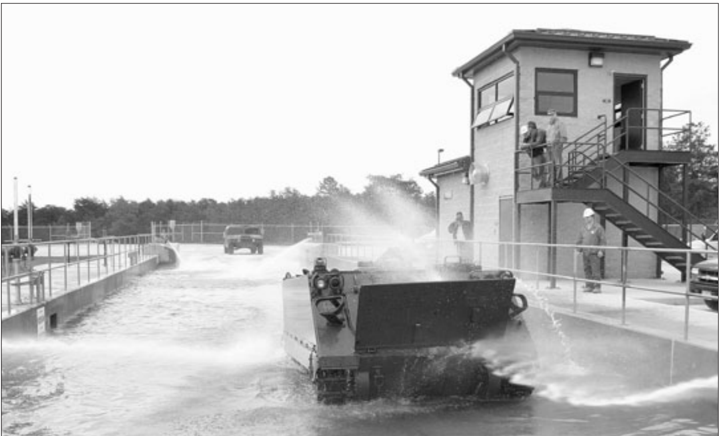
An armored personnel carrier proceeds through Fort Dix's Tactical Vehicle Wash Facility
