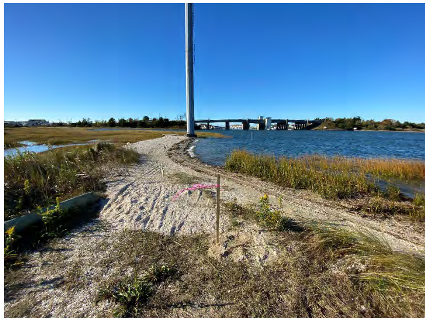
Photo #8: View from site facing southwest showing project site.
