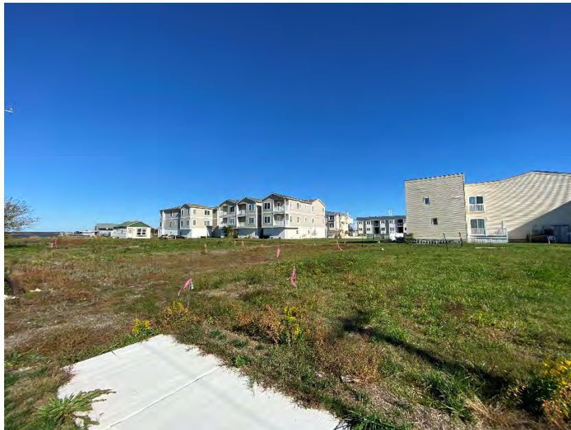
Photo #2: View from Andrews Avenue facing north showing the project site.
