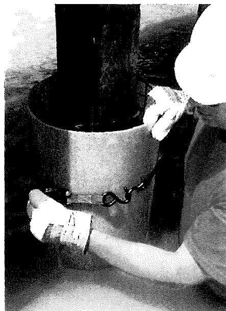
Grout can be pumped as soon as the SeaShield Fiber-Form jacket is secured in place.
